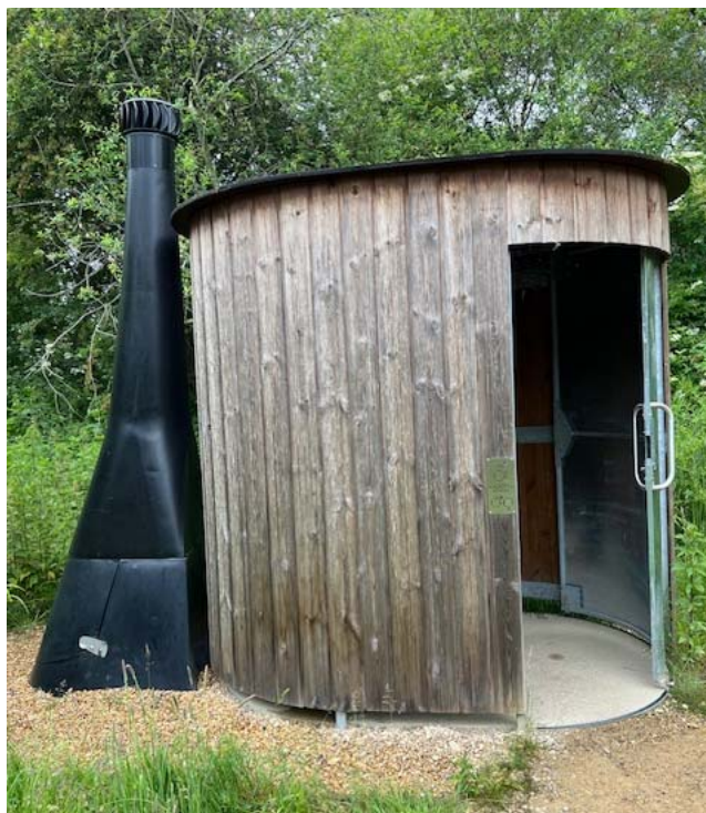
Example of Kazuba Toilet at RSPB Fowlmere
