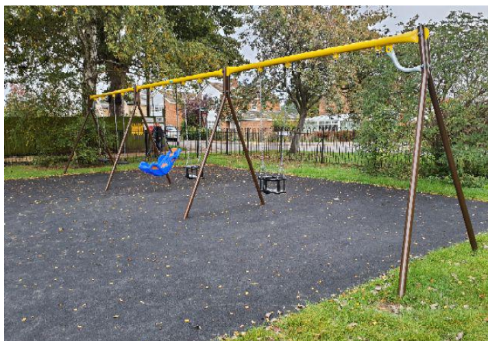
Finding: The end seat has gone and requires replacing
