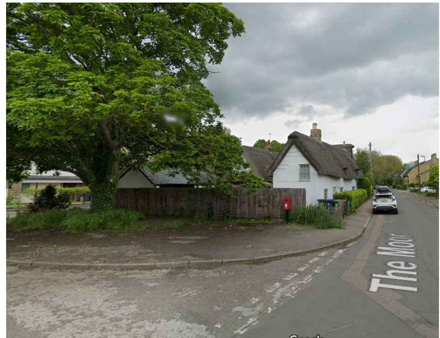
2023 shows sign missing
