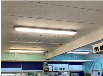
Figure 3: Example of RAAC in flat roofs and floors
