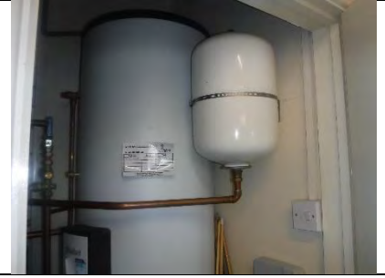
CYLINDER 1 EXPANSION VESSEL FIT FLUSHING VALVE
