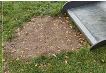
Finding: The grass has eroded within the impact area of the Action: Reinstate the grass or provide an all weather equipment and may not provide the necessary impact attenuating properties for the equipment fall height; the surface may also be slippery in wet weather
