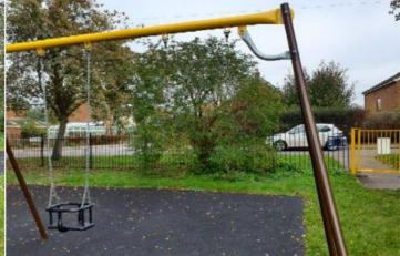
**Finding:** The seat(s) and suspension were missing at the time of inspection and the inspector was unable to make a full compliance assessment
