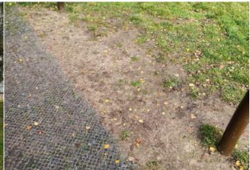
Finding: The grass has eroded within the impact area of the Action: Reinstate the grass or provide an all weather equipment and may not provide the necessary impact surface attenuating properties for the equipment fall height; the
