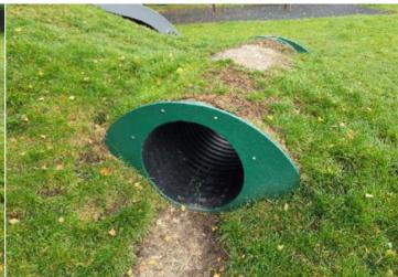
Finding: This design / configuration of tunnel mound is well established and has been successfully included in large quantities of playgrounds throughout the UK. Whilst the design does not fully meet the requirements of BS EN 1176 with regards to falls in excess of 600mm over the edge of the tunnel to the surface below, it has been risk assessed as fit for purpose in this regard and no changes are recommended to the design unless otherwise stated in additional findings
