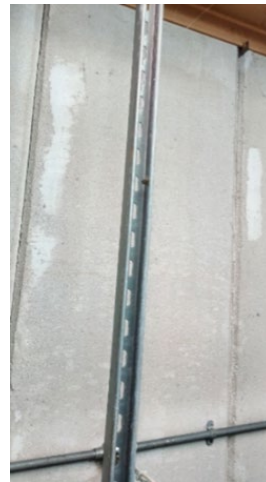
Figure 9: V-shaped grooves at 600mm spacing
