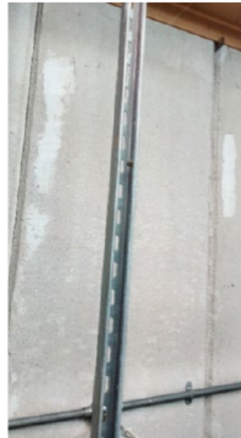
Figure 9: V-shaped grooves at 600mm spacing
