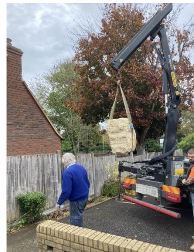
Crane lifting the boulder in place
