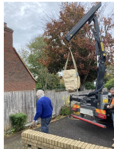
Crane lifting the boulder in place
