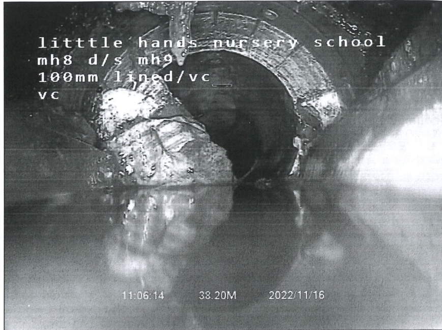
MH8 X_1f7c8b90-19ca-4ab0-8fa6-d101678ba8f3_20221117_141009_198.jpg, 00:01:45, 38.30 m Finish node, manhole, reference: MH9, BURIED MANHOLE
