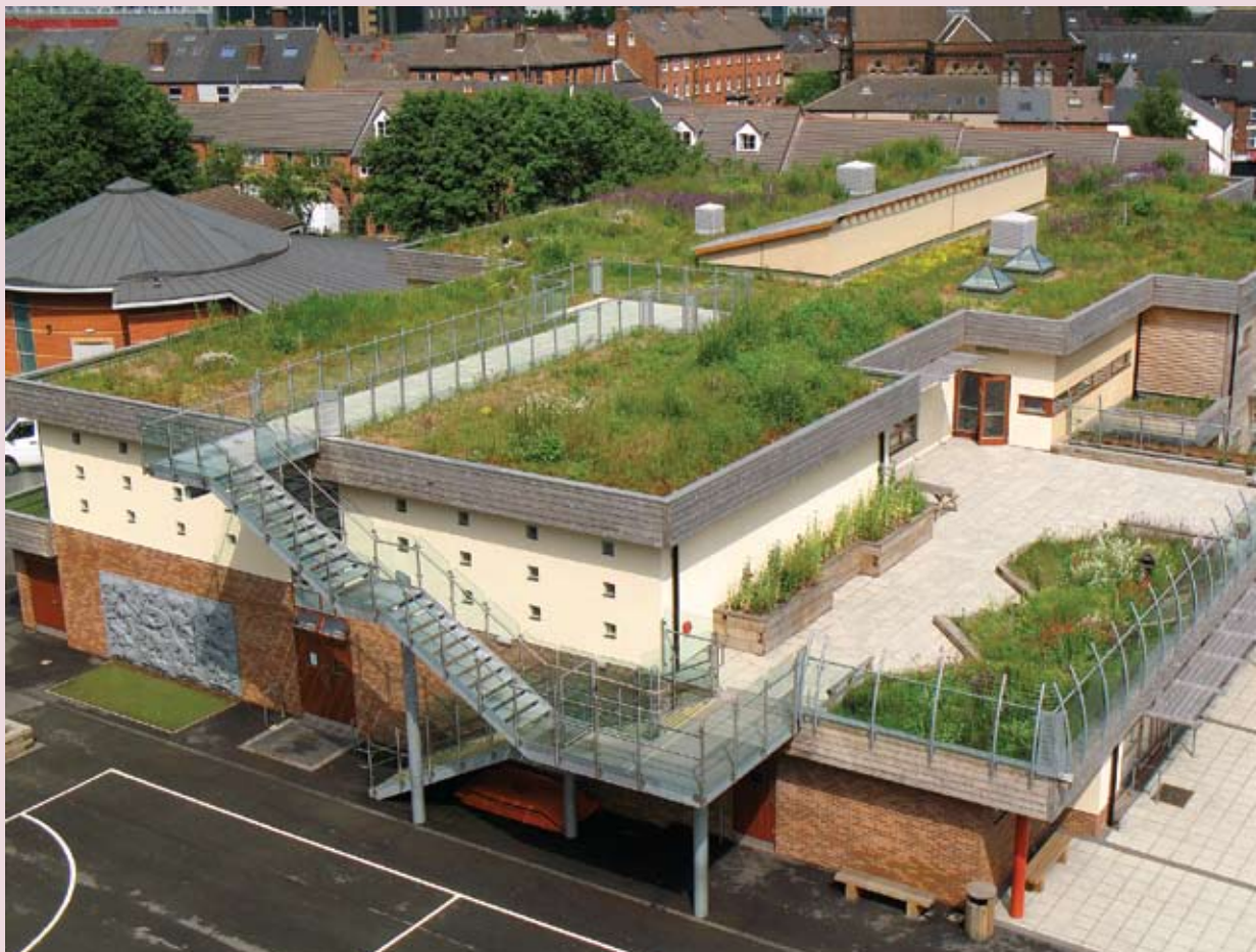
© Sheffield Green Roof Centre
