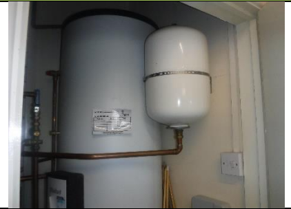
Cylinder 1 expansion vessel fit flushing valve
