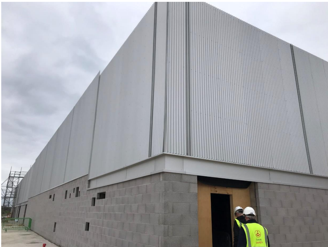
Figure 2 – Tech Barn Sinusoidal cladding and blockwork
