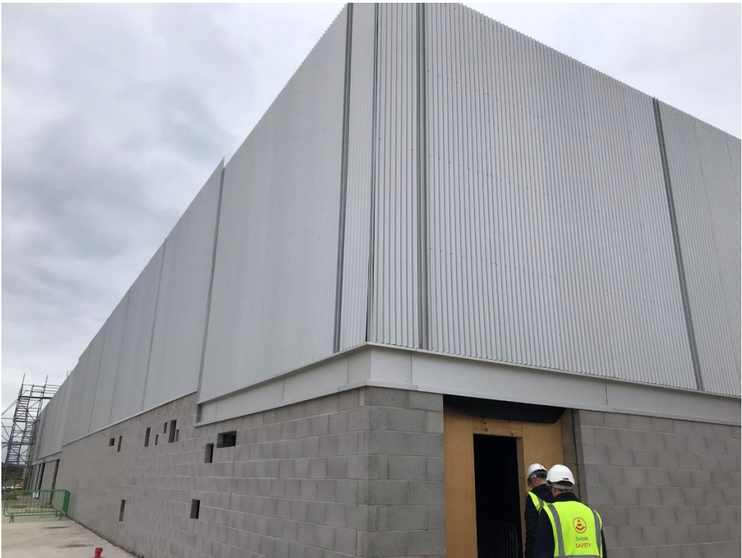
Figure 2 – Tech Barn Sinusoidal cladding and blockwork
