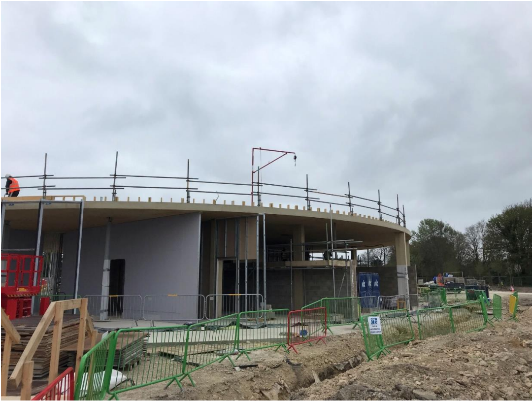
Figure 1 – Block work and Partitioning commencing inside the Forum Building
