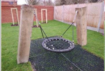
**Finding:** Swings of this design should have a secondary safety device fitted to prevent collapse of the seat in the event of a joint failure to meet the requirements of BS EN 1176 Part 2. NOTE - this is due to the pivot height being marginally over 1.30m (1.35m) as this requirement is not valid for pivots under 1.30m
