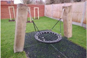
**Finding:** The seat clearance from finished surface level to the underside of the seat is too low at 60mm when measured in its most onerous position and does not meet the requirements of BS EN 1176 Part 2
