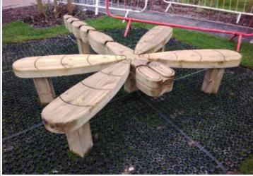
Finding: The tree forms a hard object within the falling space of the equipment in contravention of the requirements of BS EN 1176 Part 1 (Distance required 1.50m / Provided 1.02m)
