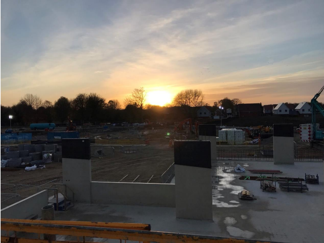
Figure 3 – View from the Hive Roof
