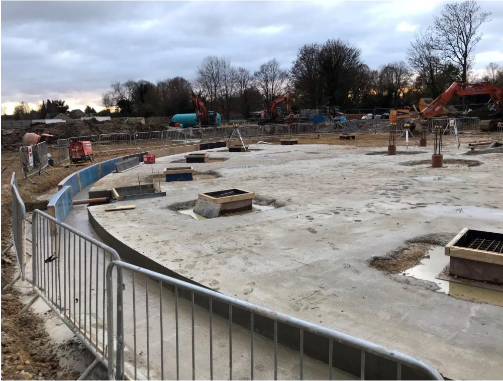
Figure 1 – The Start of the Forum Foundations
