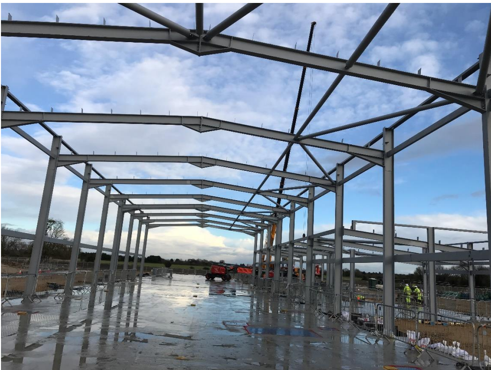
Figure 2 – The Tech Barn Steel Frame
