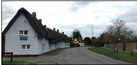
Left: View looking west along Melbourn High Street at the entrance to the Conservation Area with Sheepshead Row on the left, and the tall brick and flint wall forming a sense of enclosure on the right.
