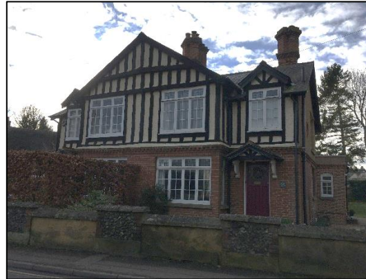
Above: An Edwardian example of semi-detached dwellings with brick to the ground floor and render with decorative timber framing to the upper storey, with prominent brick chimney stacks.
