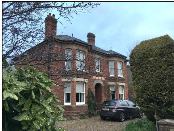
Left: A fine example of a late 19 th century detached villa, constructed of brick with symmetrical frontage comprising double-height bay windows and timber vertical sliding sashes. The door is recessed, under an arched lintel and the windows feature flat moulded stone lintels.
