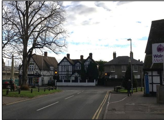
Above: A group of buildings, one timber framed and rendered with clay tile roof, the middle unit mirrors this detail with a clay tile roof and Arts and Crafts decorative false timber framing.
