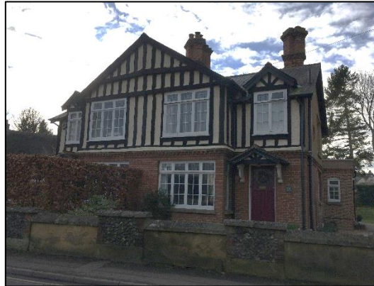
Above: An Edwardian example of semi-detached dwellings with brick to the ground floor and render with decorative timber framing to the upper storey, with prominent brick chimney stacks.
