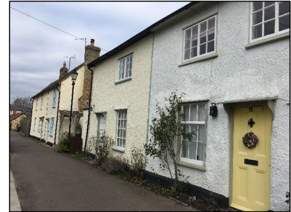
Above: Example of semi-detached 'cottages' of two storeys, with rendered walls and timber windows; larger sash-style to the ground floor and side-hung casement above. The doors are timber panelled with small hood canopy's over, on simple brackets.
