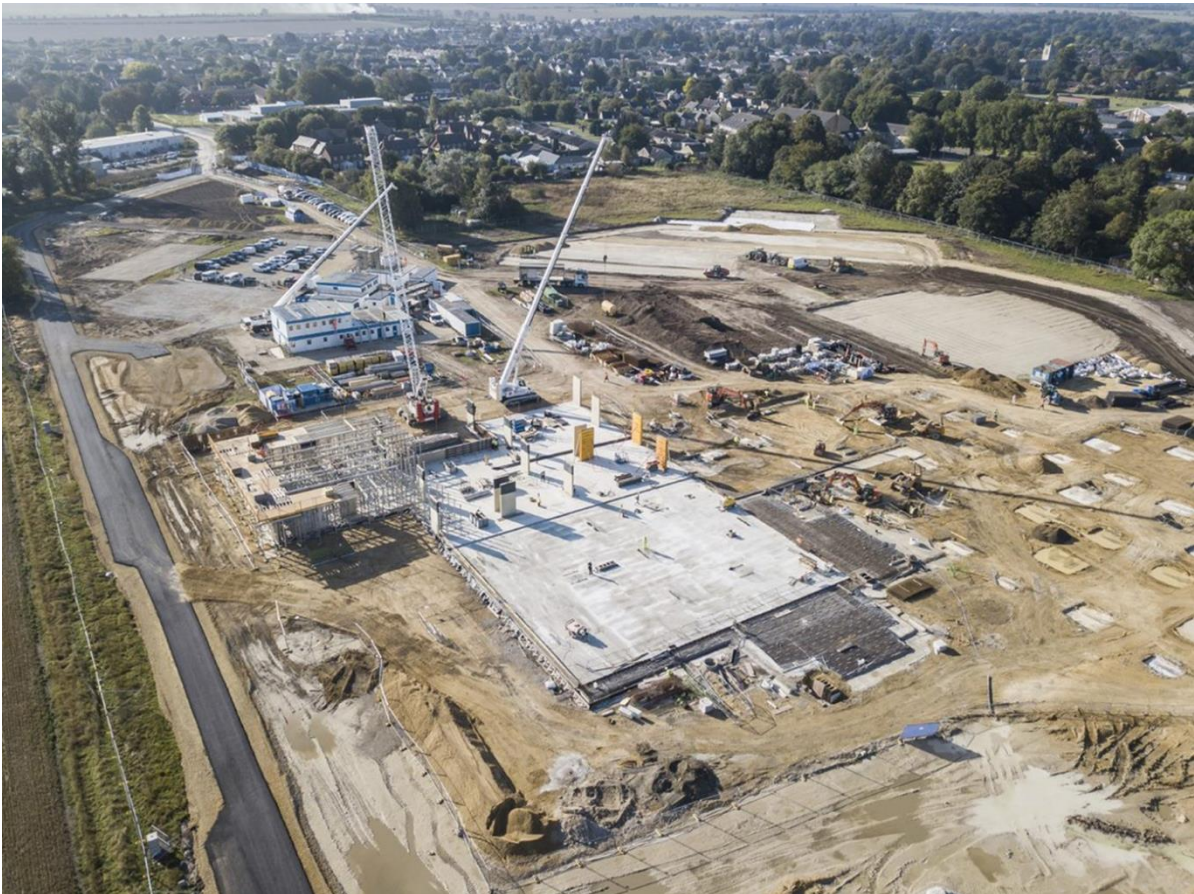
Figure 7 – Aerial Photo 24 th September
