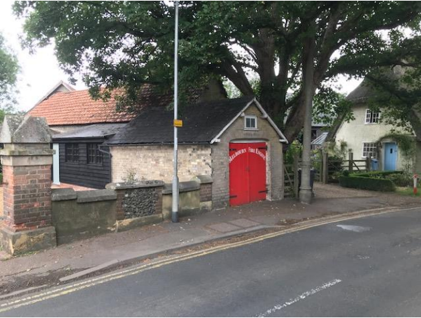
Old Fire Station
