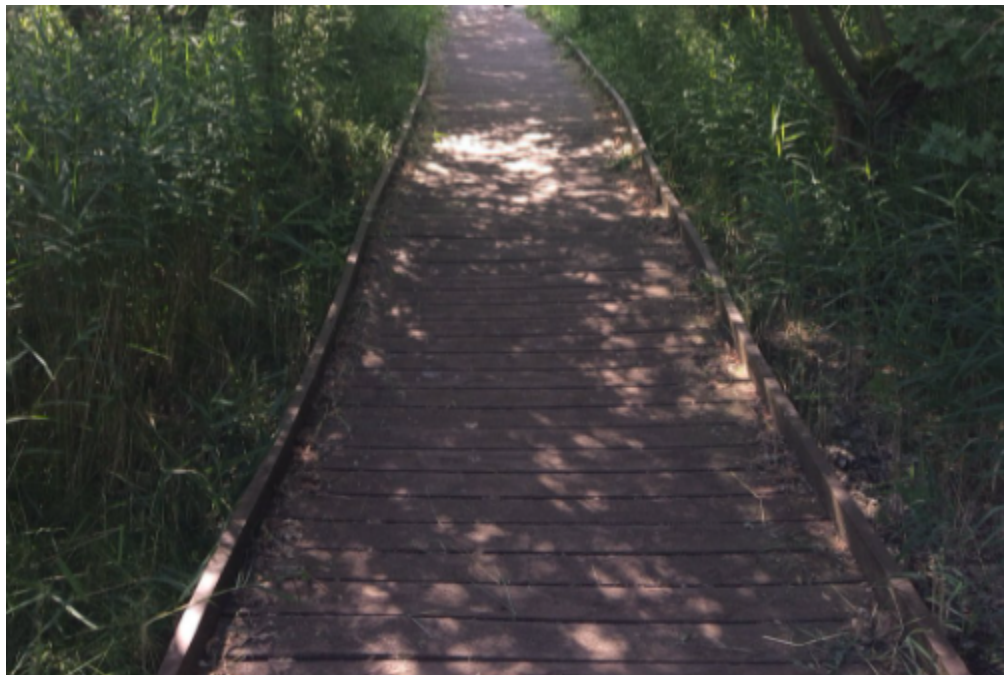
Example of low level boardwalk without handrail.
