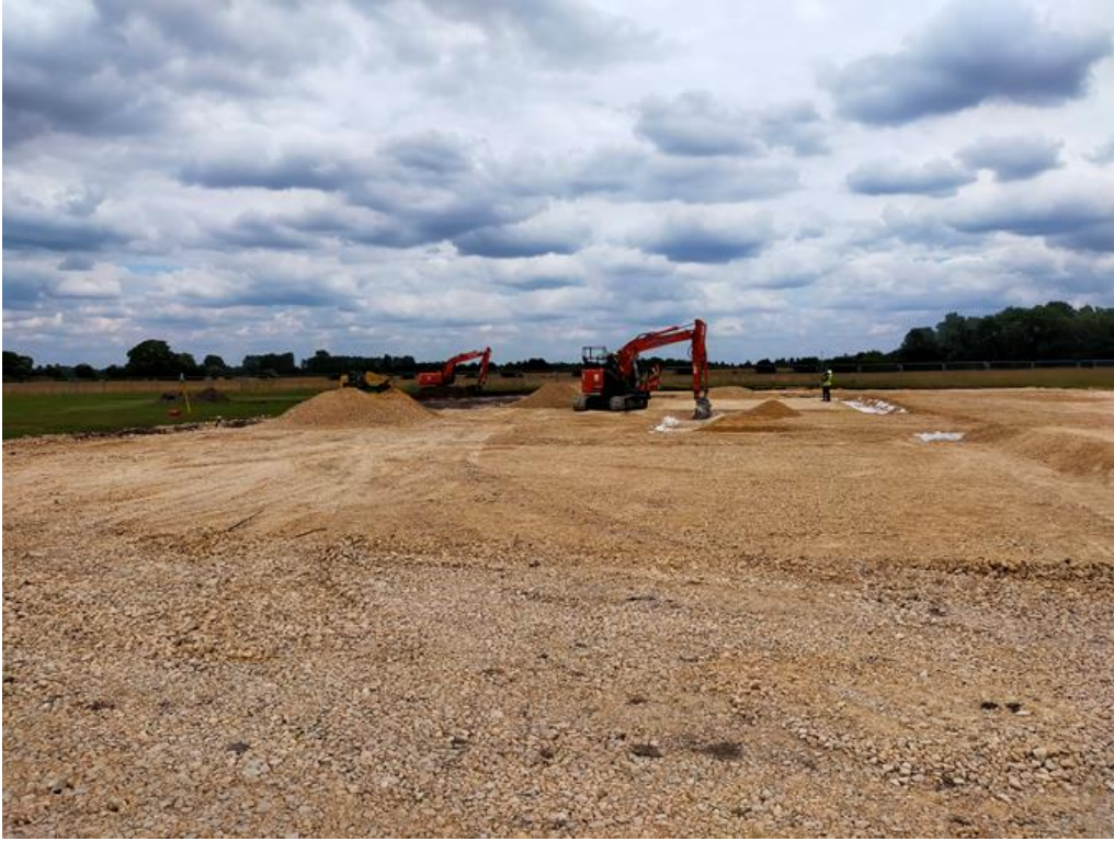
Figure 1 – Clearance and construction of The Hive building sub base
