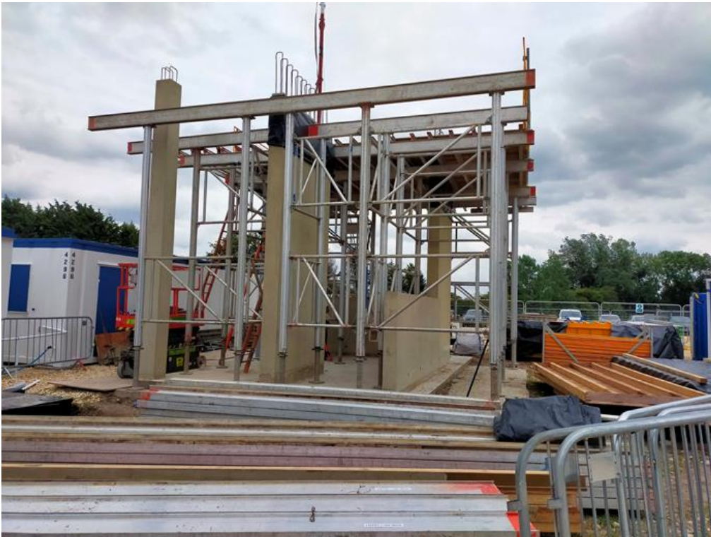
Figure 2 - Concrete columns - mock up 'prototype'
