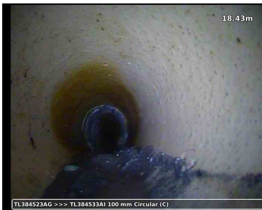
20210617-185600-snap0023.jpg, 00:04:41, 18.43 m Crack, circumferential, from 07 to 05 o'clock
