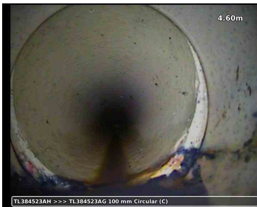
20210617-184209-snap0003.jpg, 00:00:53, 4.60 m Joint displaced, medium
