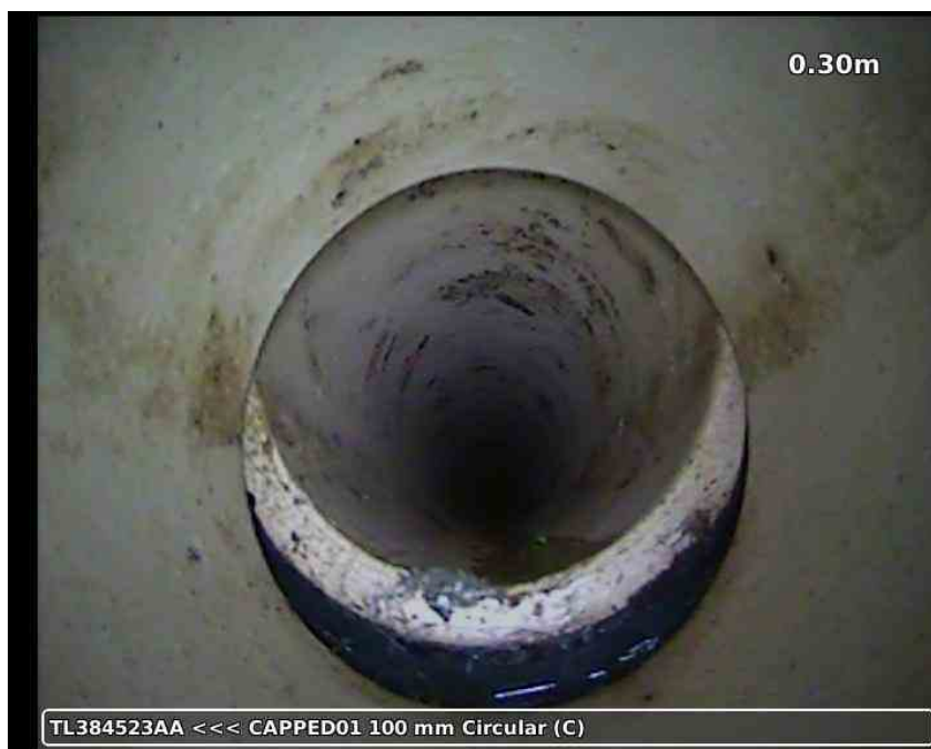
20210617-161651-snap0002.jpg, 00:00:18, 0.30 m Joint displaced, 20 mm displacement
