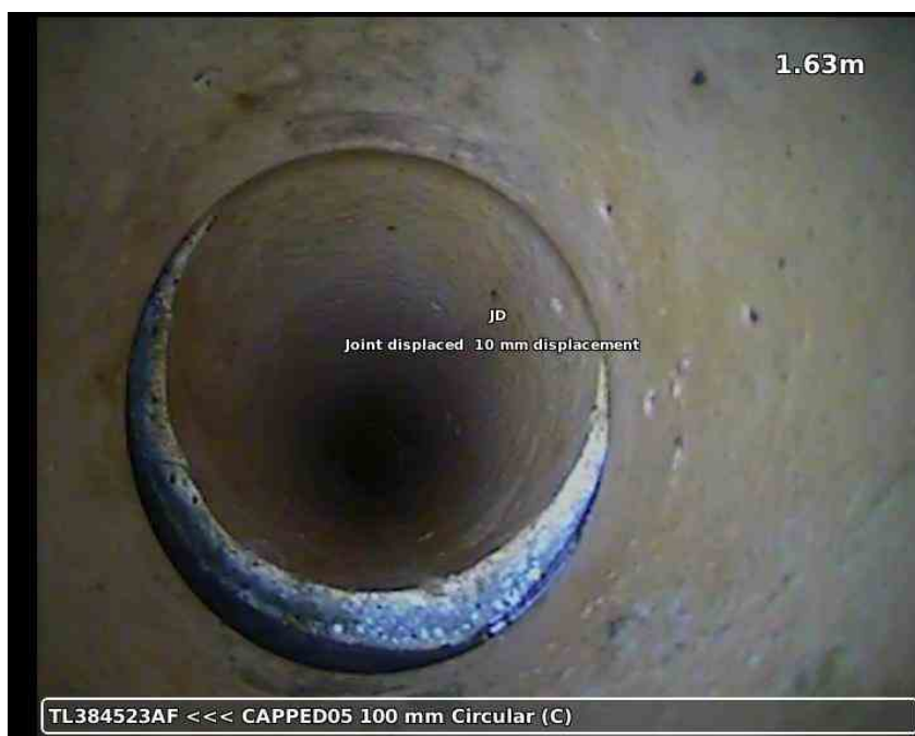
20210617-180419-snap0003.jpg, 00:00:40, 1.63 m Open joint, medium
