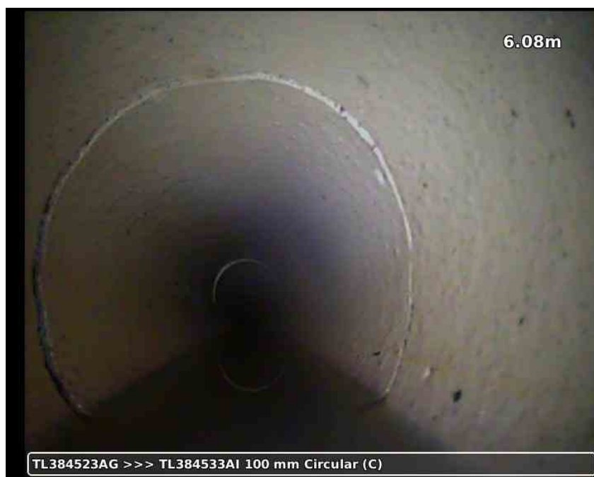
20210617-185600-snap0009.jpg, 00:02:01, 6.08 m Fracture, circumferential, from 07 to 05 o'clock
