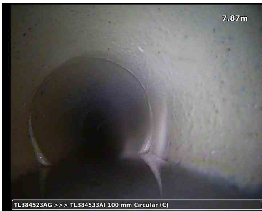
20210617-185600-snap0012.jpg, 00:02:36, 7.87 m Joint displaced, medium
