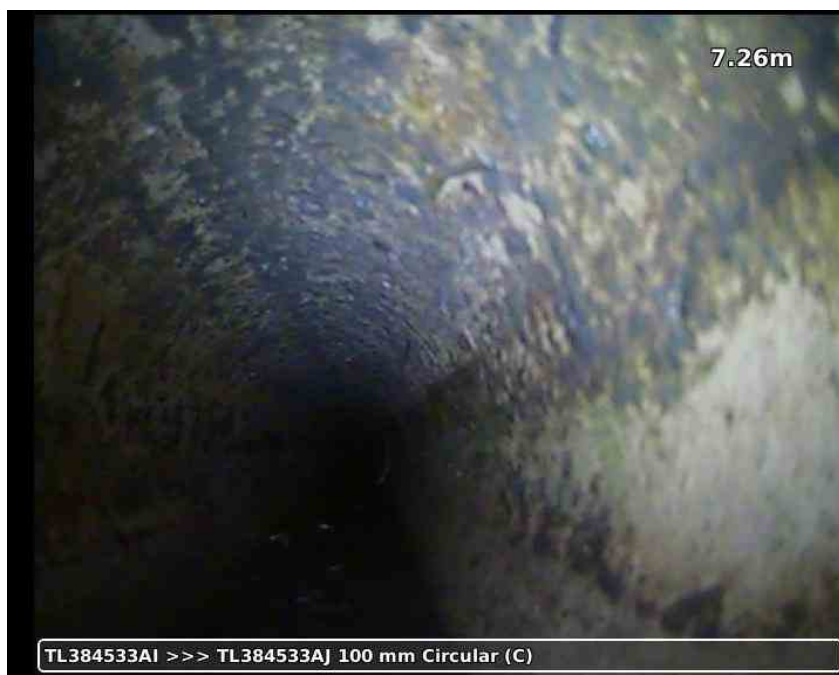
20210617-191337-snap0010.jpg, 00:02:38, 7.26 m Attached deposits, fouling, from 07 to 05 o'clock, 5% % cross-sectional area loss, S02
