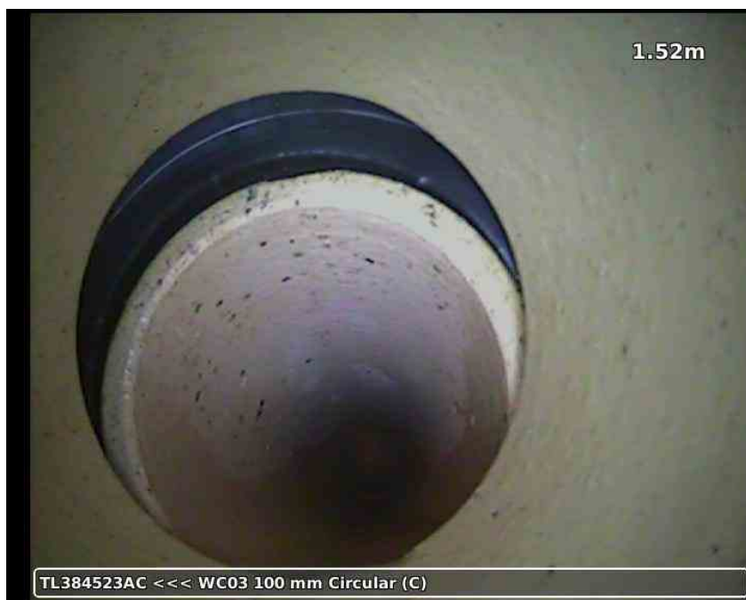
20210617-171046-snap0002.jpg, 00:00:23, 1.52 m Open joint, large
