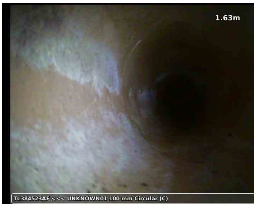
20210617-175837-snap0003.jpg, 00:00:41, 1.63 m Fracture, circumferential, from 03 to 11 o'clock
