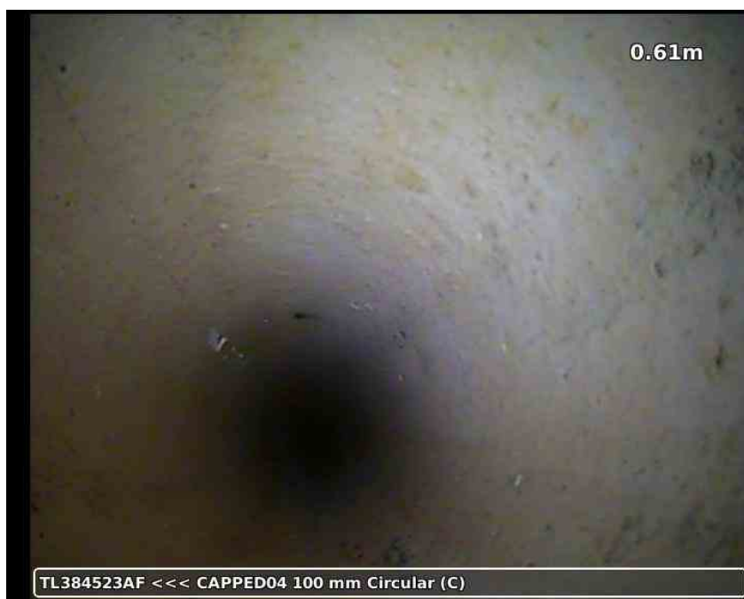
20210617-180144-snap0003.jpg, 00:00:35, 0.61 m Fracture, longitudinal, at 11 o'clock, S01
