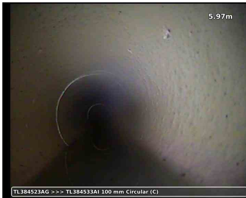
20210617-185600-snap0008.jpg, 00:01:41, 5.97 m Water level, 20% % of the vertical dimension
