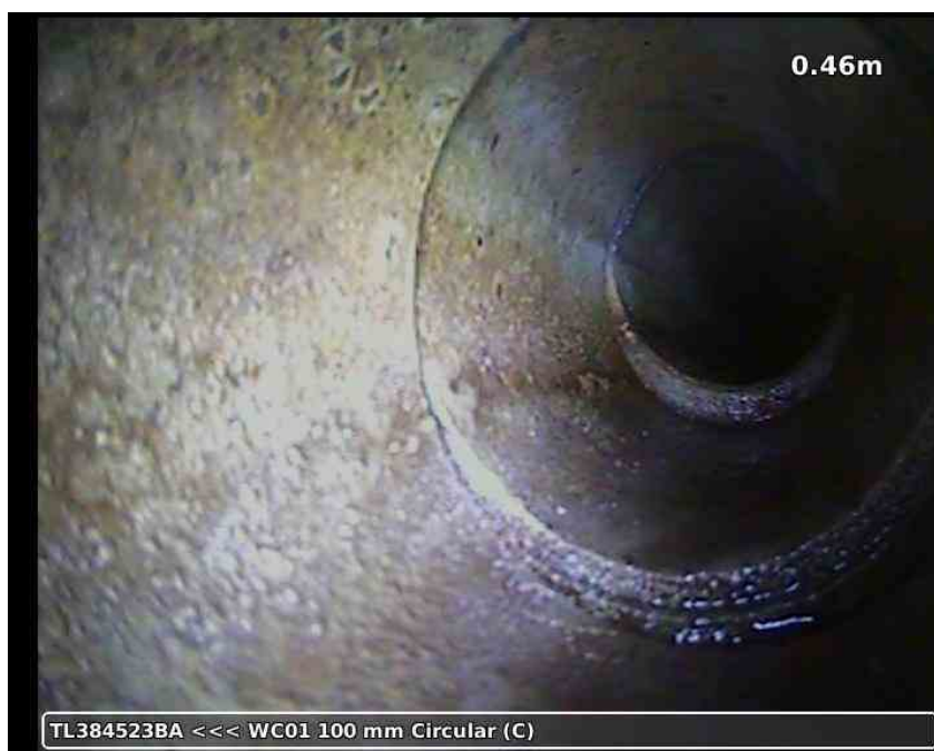
20210617-164432-snap0005.jpg, 00:00:35, 0.46 m Open joint, medium
