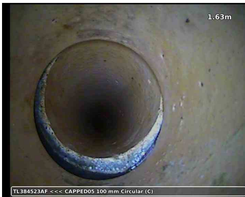
20210617-180419-snap0002.jpg, 00:00:34, 1.63 m Joint displaced, 10 mm displacement
