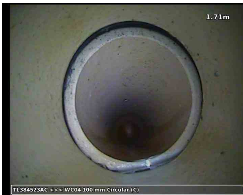
20210617-171300-snap0003.jpg, 00:00:29, 1.71 m Open joint, medium
