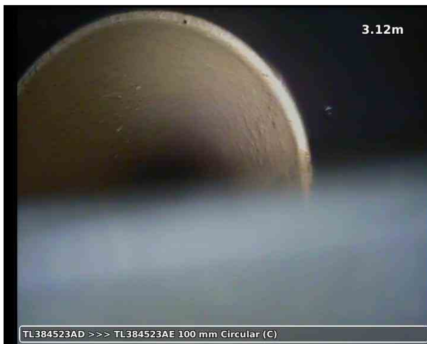
20210617-173215-snap0004.jpg, 00:01:18, 3.12 m Material changes to vitrified clay
