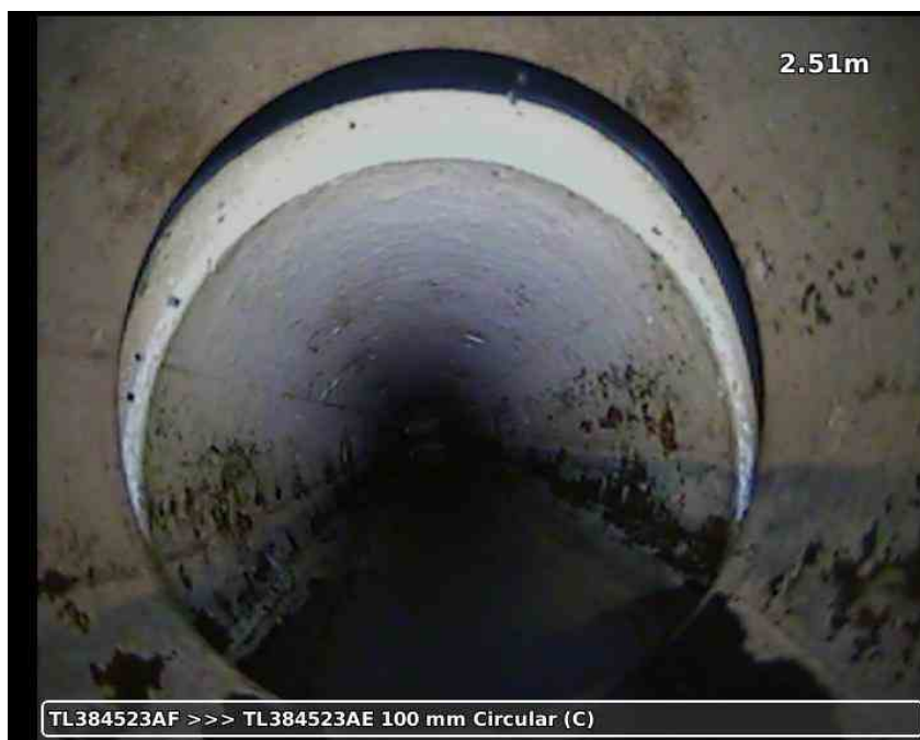
20210617-180721-snap0002.jpg, 00:00:46, 2.51 m Joint displaced, 20 mm displacement
