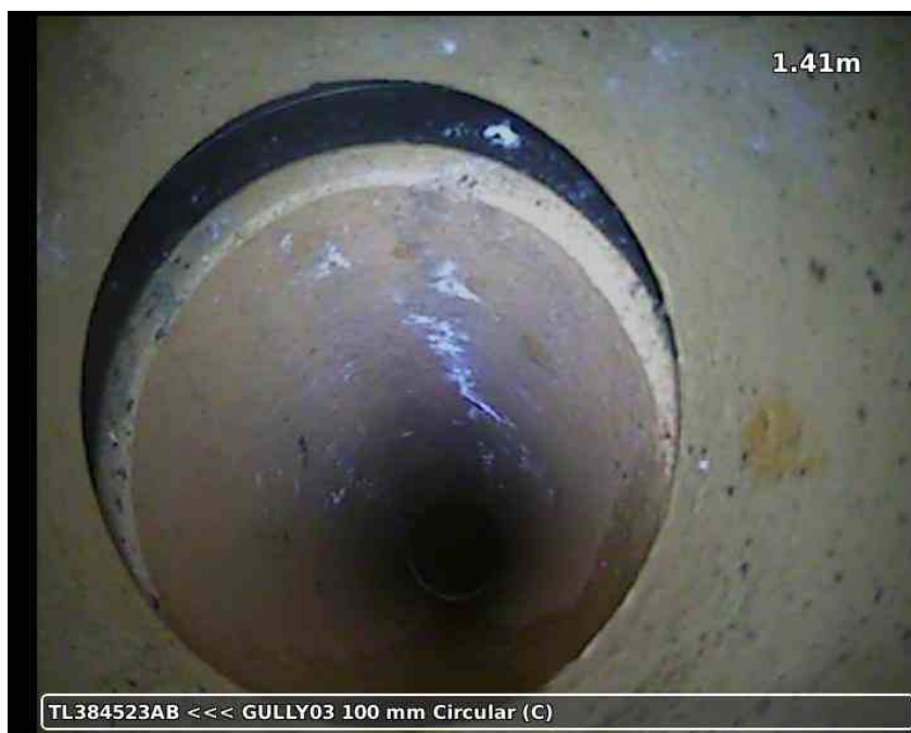
20210617-165624-snap0002.jpg, 00:00:24, 1.41 m Joint displaced, 20 mm displacement
