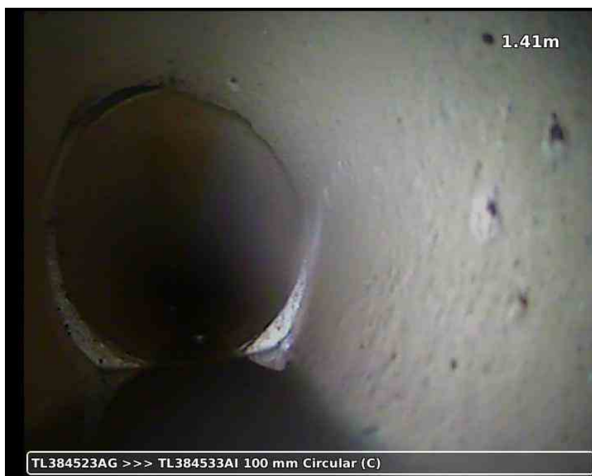
20210617-185600-snap0005.jpg, 00:00:45, 1.41 m Joint displaced, medium
