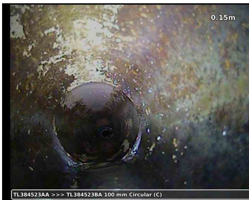
20210617-163005-snap0003.jpg, 00:00:25, 0.15 m Attached deposits, fouling, from 01 to 11 o'clock, 5% % cross-sectional area loss, S01
