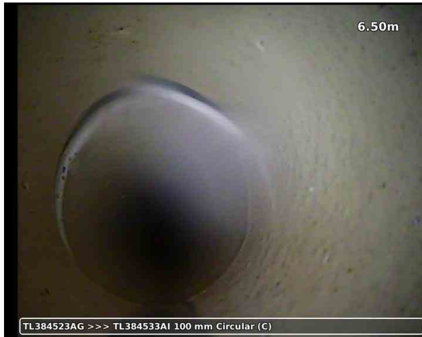
20210617-185600-snap0010.jpg, 00:02:16, 6.50 m Joint displaced, medium
