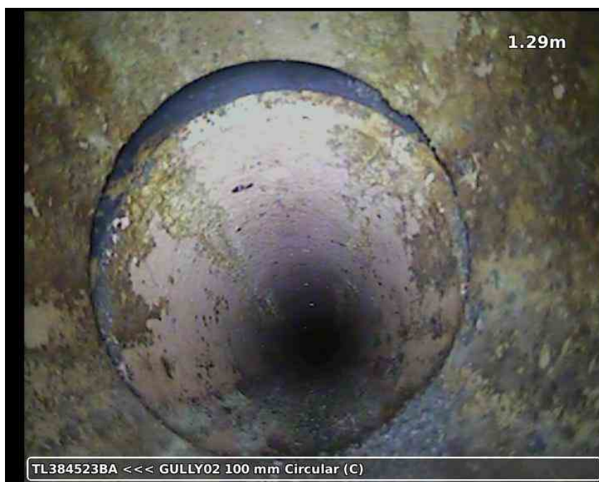
20210617-164707-snap0003.jpg, 00:00:35, 1.29 m Open joint, medium
