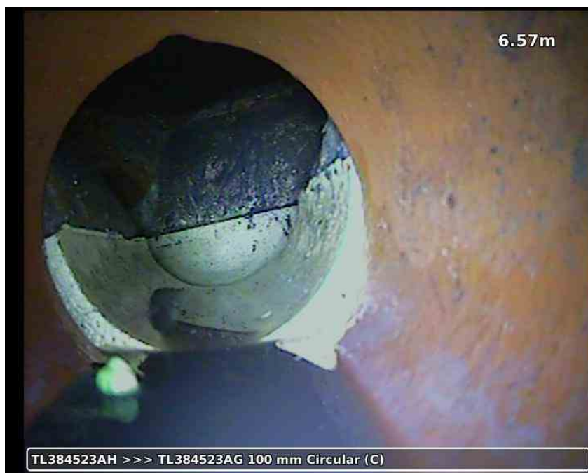
20210617-184209-snap0006.jpg, 00:01:30, 6.57 m Joint displaced, 10 mm displacement
