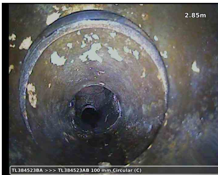
20210617-164942-snap0007.jpg, 00:01:15, 2.85 m Joint displaced, 10 mm displacement
