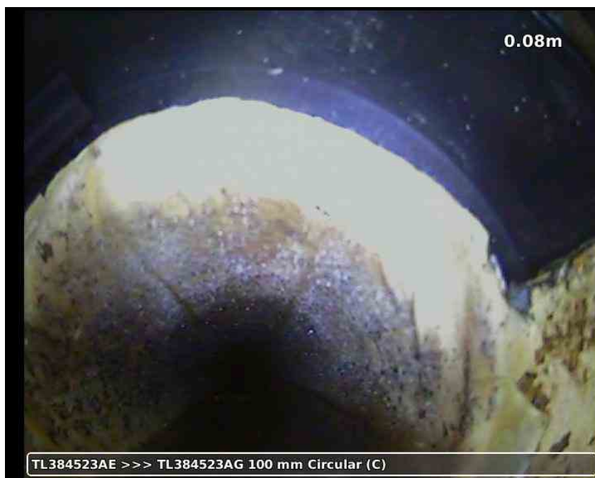
20210617-181934-snap0002.jpg, 00:00:16, 0.08 m Lining of drain or sewer with cured-in-place lining changes to polyester at this point
