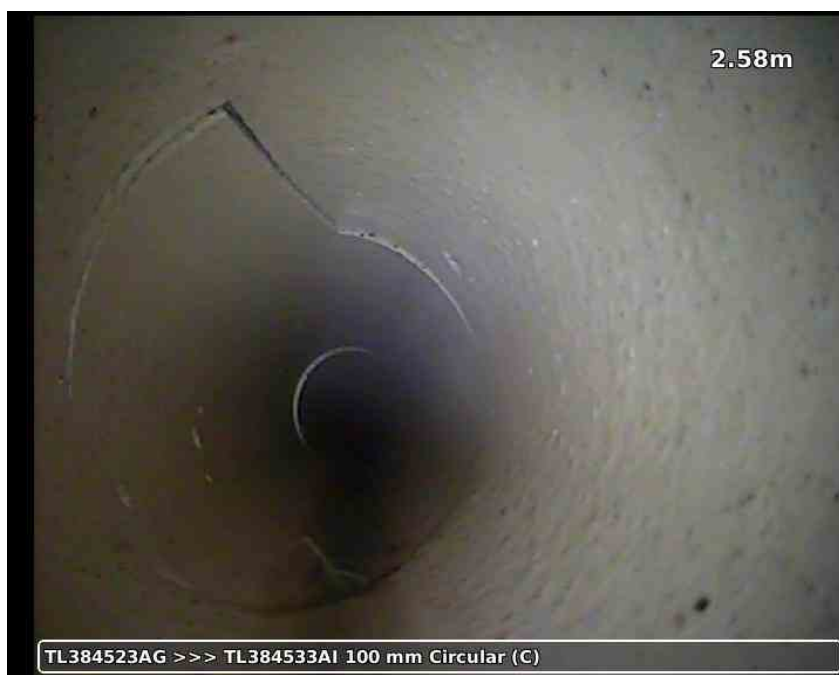
20210617-185600-snap0007.jpg, 00:01:12, 2.58 m Fracture spiral, from 12 to 11 o'clock
