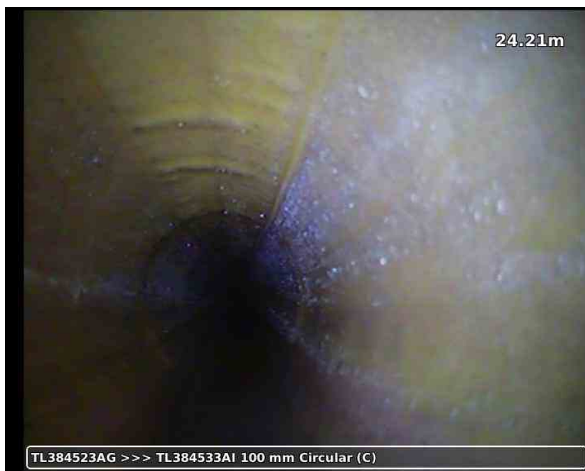
20210617-185600-snap0026.jpg, 00:05:49, 24.21 m Water level, 15% % of the vertical dimension
