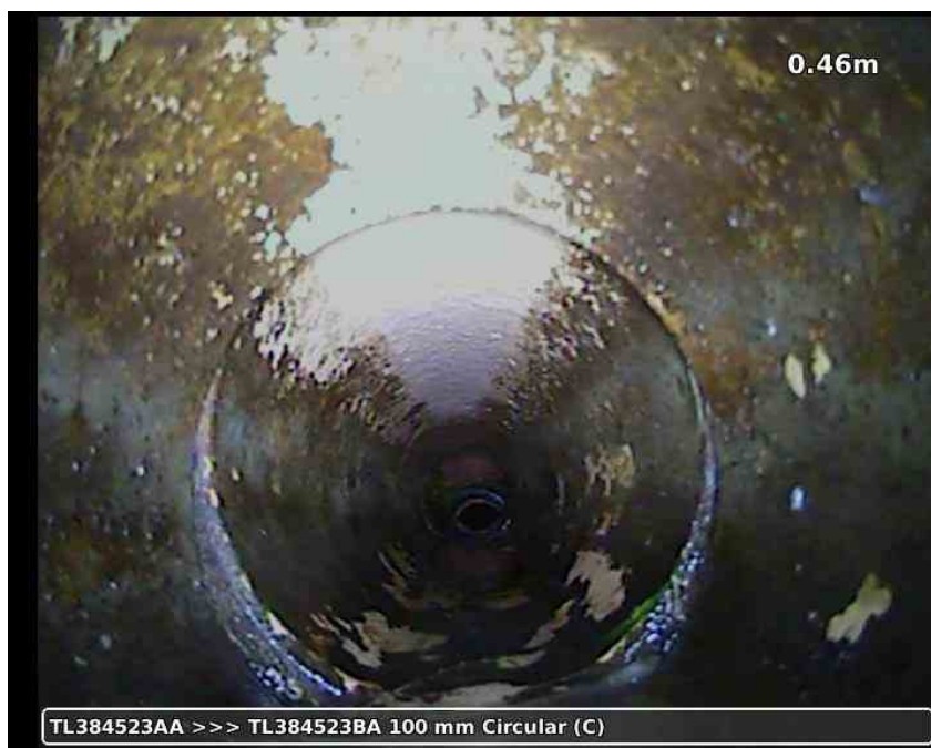
20210617-163005-snap0004.jpg, 00:00:39, 0.46 m Joint displaced, medium
