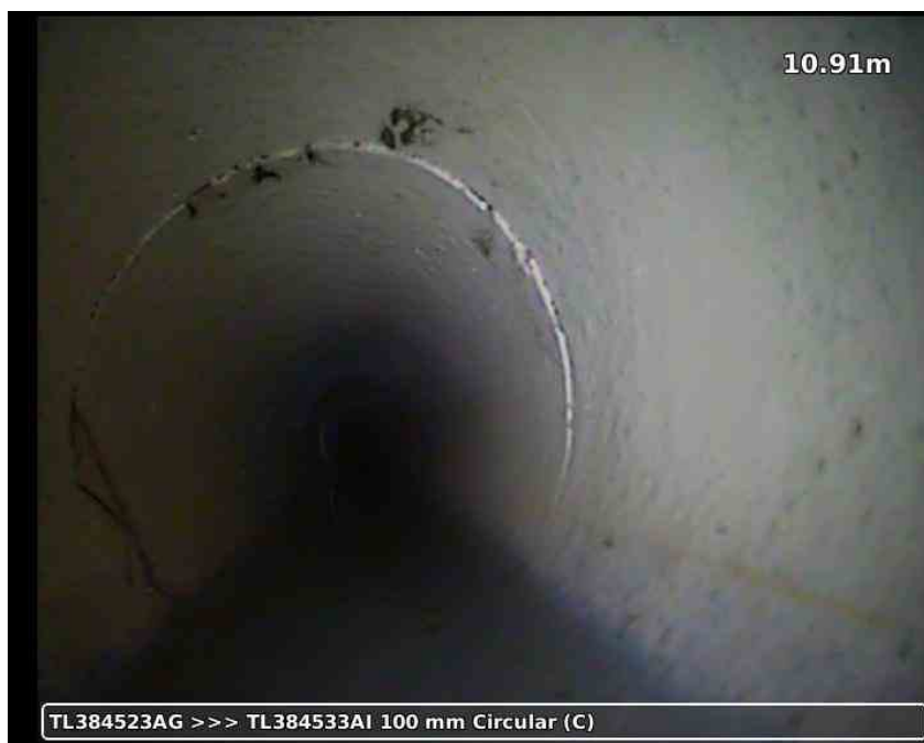
20210617-185600-snap0016.jpg, 00:03:14, 10.91 m Fracture, circumferential, from 07 to 05 o'clock
