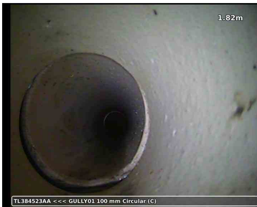
20210617-161336-snap0004.jpg, 00:00:31, 1.82 m Open joint, medium
