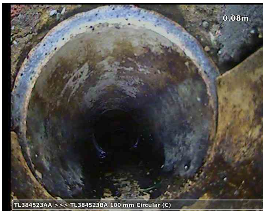
20210617-163005-snap0002.jpg, 00:00:17, 0.08 m Joint displaced, medium
