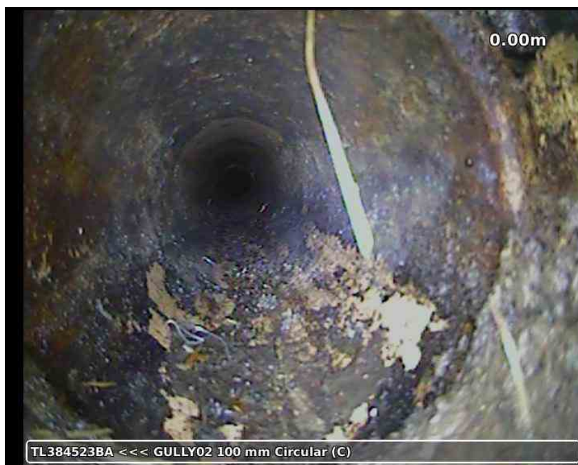
20210617-164707-snap0002.jpg, 00:00:12, 0.00 m Attached deposits, fouling, from 01 to 12 o'clock, 5% % cross-sectional area loss, S01
