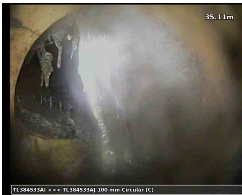
20210617-191337-snap0025.jpg, 00:08:34, 35.11 m Roots, mass, 30% % cross-sectional area loss
