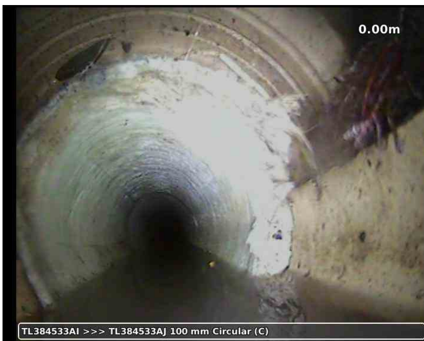
20210617-191337-snap0002.jpg, 00:00:19, 0.00 m Lining of drain or sewer with cured-in-place lining changes to epoxy at this point
