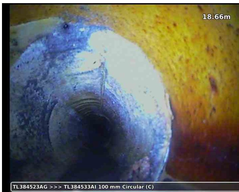
20210617-185600-snap0025.jpg, 00:04:58, 18.66 m Lining of drain or sewer with cured-in-place lining changes to polyester at this point
