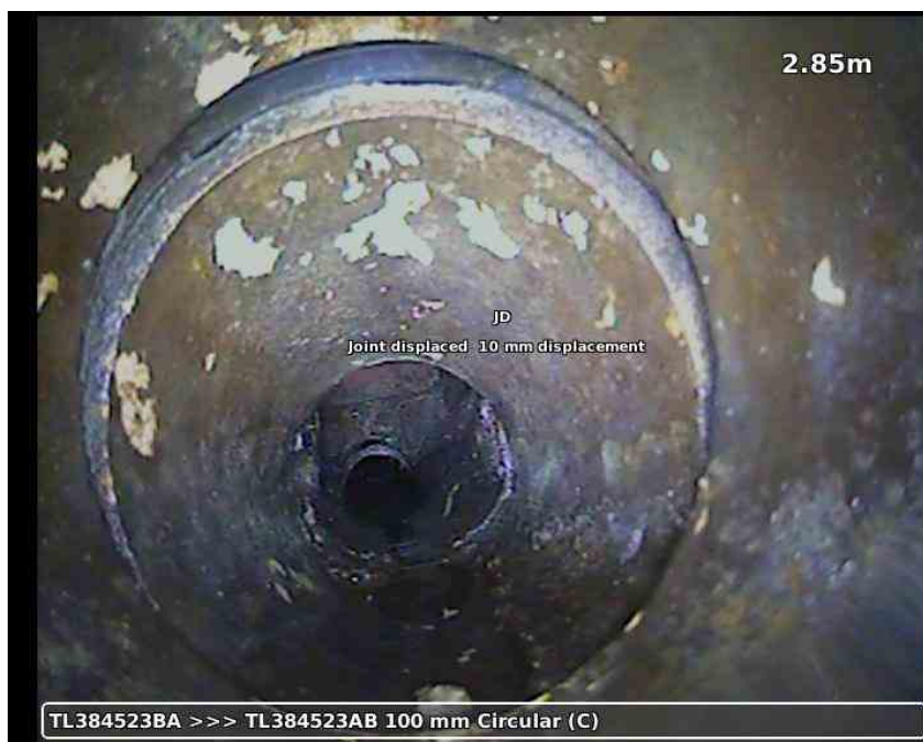
20210617-164942-snap0008.jpg, 00:01:21, 2.85 m Open joint, medium
