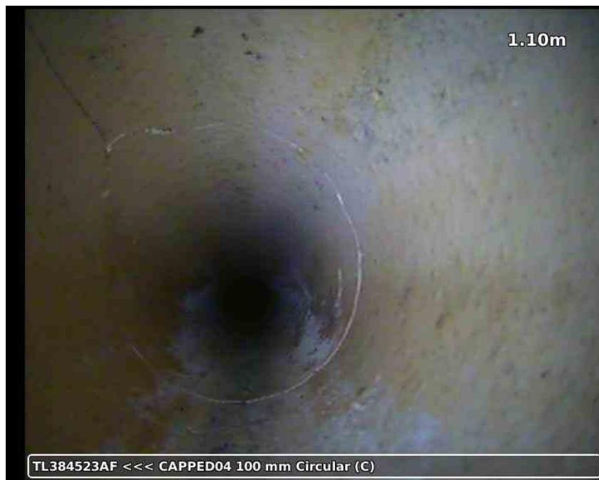
20210617-180144-snap0004.jpg, 00:00:50, 1.10 m Fracture, circumferential, from 11 to 10 o'clock
