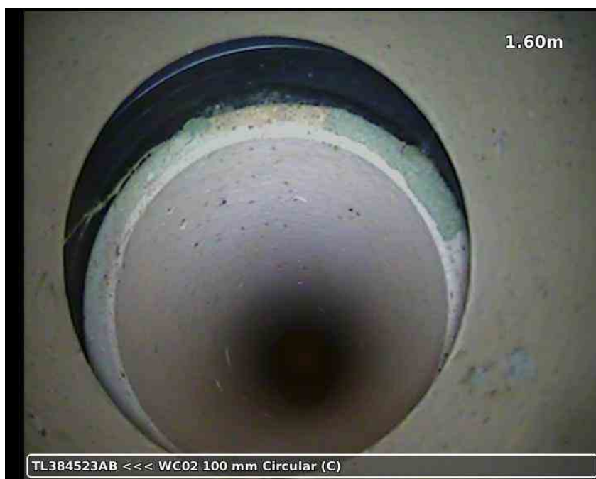
20210617-165855-snap0003.jpg, 00:00:36, 1.60 m Open joint, large
