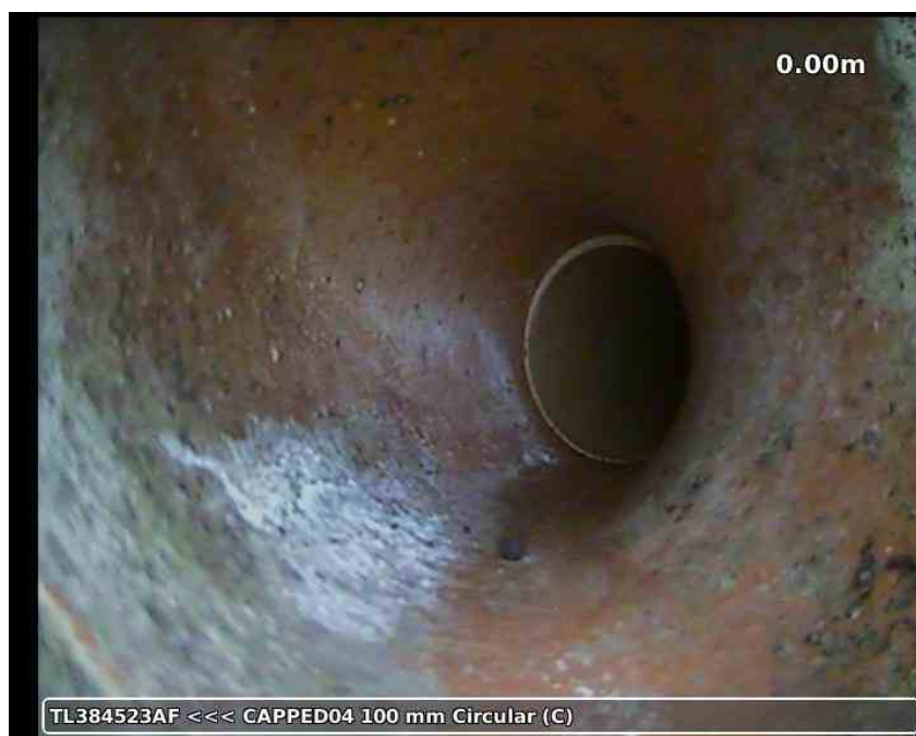
20210617-180144-snap0001.jpg, 00:00:01, 0.00 m Water level, 0% % of the vertical dimension, CAPPED OFF
