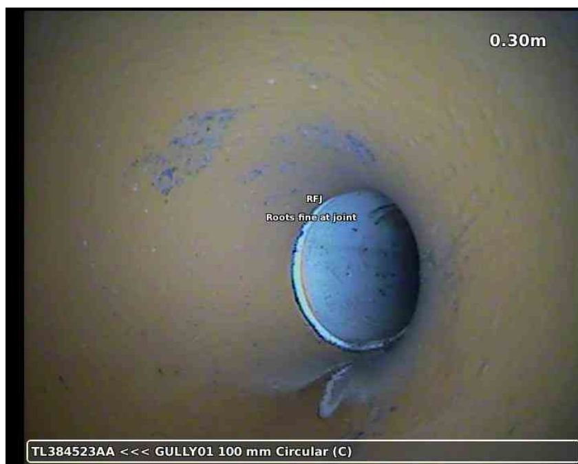
20210617-161336-snap0003.jpg, 00:00:17, 0.30 m Line deviates right
