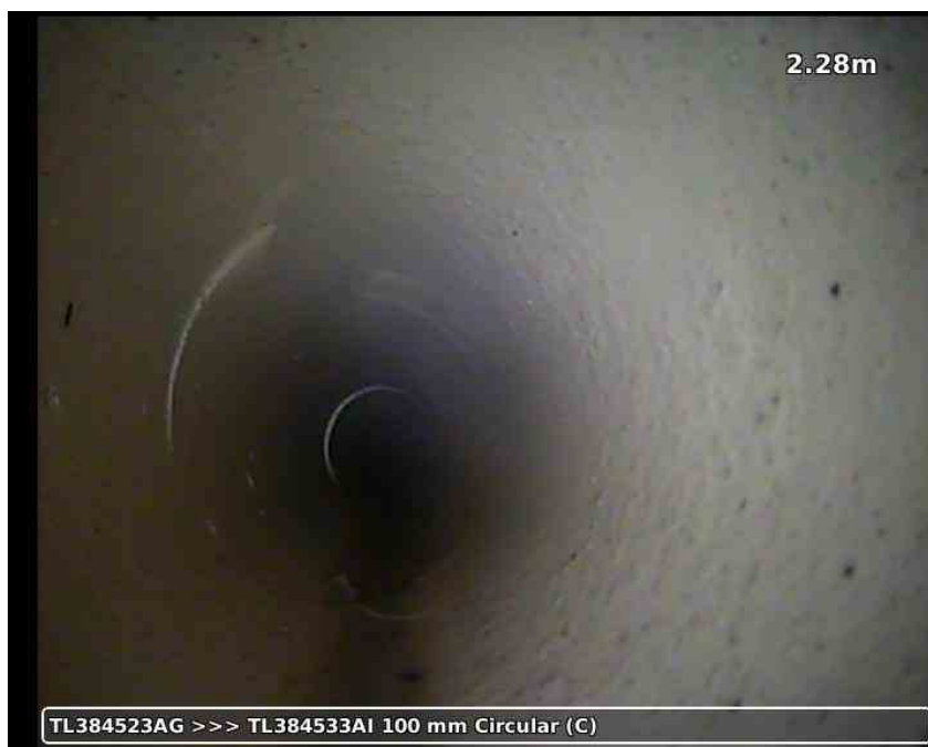
20210617-185600-snap0006.jpg, 00:01:02, 2.28 m Fracture, longitudinal, at 11 o'clock
