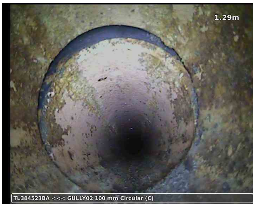
20210617-164707-snap0004.jpg, 00:00:39, 1.29 m Joint displaced, 10 mm displacement
