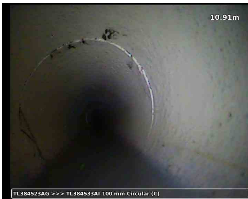
20210617-185600-snap0017.jpg, 00:03:18, 10.91 m Roots, fine, ENTERING THROUGH FC
