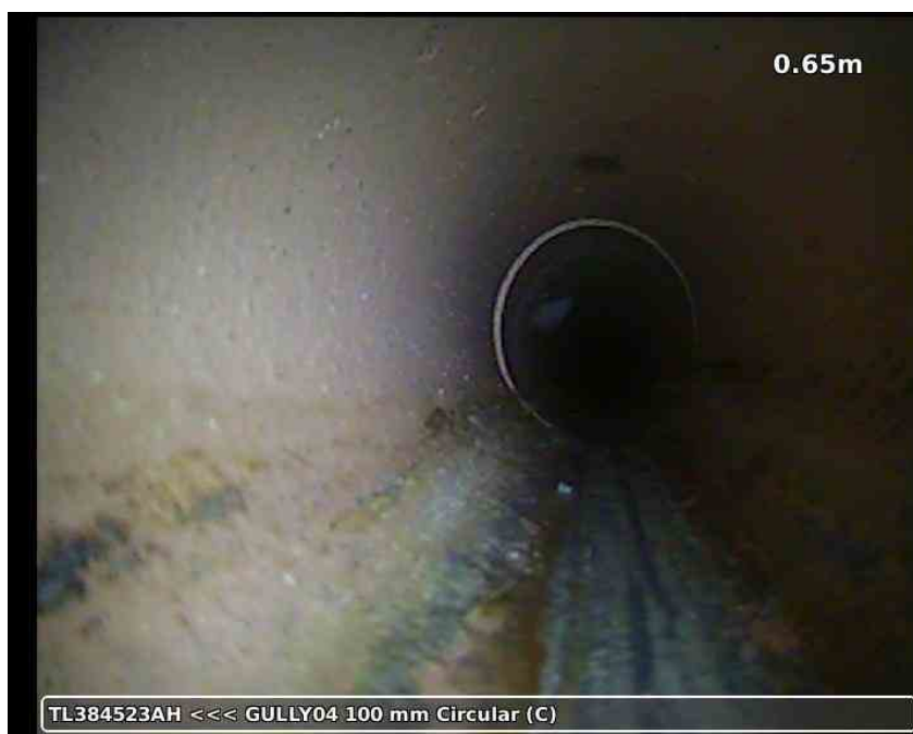
20210617-183231-snap0003.jpg, 00:00:12, 0.65 m Attached deposits, encrustation, from 05 to 07 o'clock, 5% % cross-sectional area loss, S01, Scale
