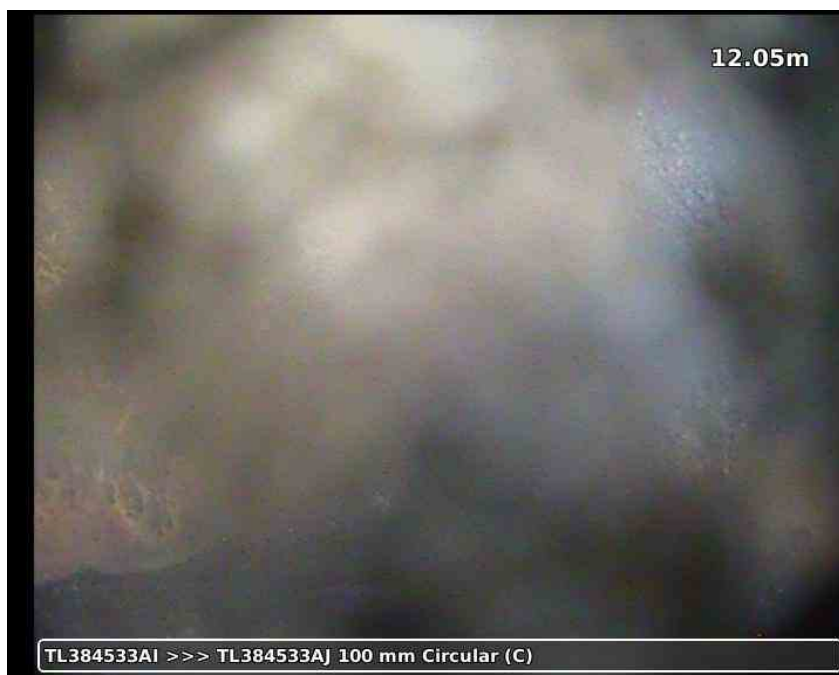
20210617-191337-snap0014.jpg, 00:04:06, 12.05 m Loss of vision, silt, S04
