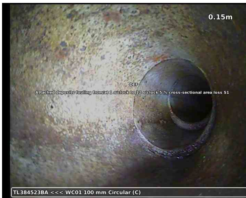
20210617-164432-snap0004.jpg, 00:00:24, 0.15 m Line deviates right
