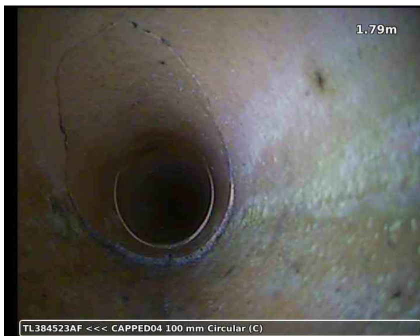
20210617-180144-snap0005.jpg, 00:01:11, 1.79 m Fracture spiral, from 12 to 11 o'clock
