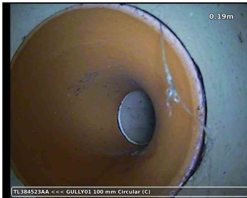
20210617-161336-snap0002.jpg, 00:00:11, 0.19 m Roots, fine at joint
