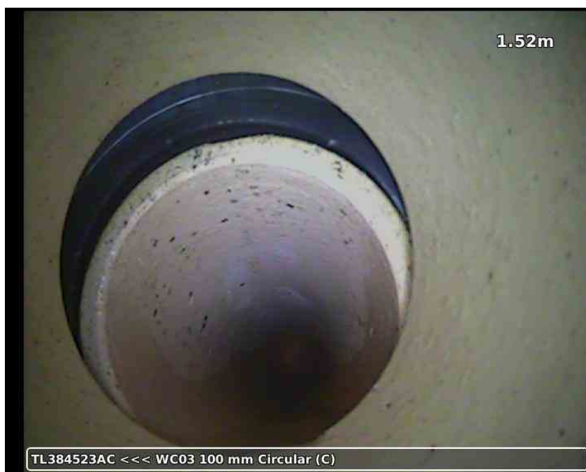
20210617-171046-snap0003.jpg, 00:00:27, 1.52 m Joint displaced, 20 mm displacement
