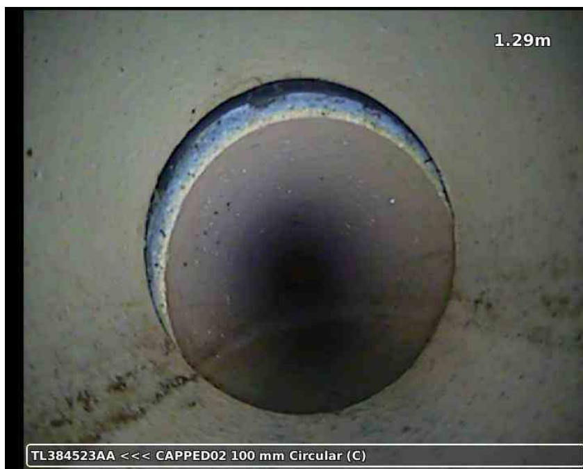
20210617-161854-snap0002.jpg, 00:00:28, 1.29 m Joint displaced, 10 mm displacement
