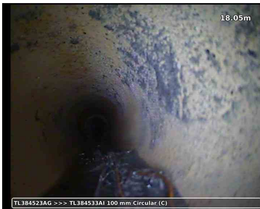
20210617-185600-snap0022.jpg, 00:04:28, 18.05 m Roots, mass, 20% % cross-sectional area loss
