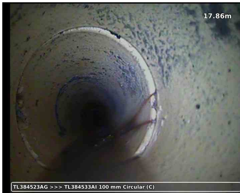
20210617-185600-snap0020.jpg, 00:04:16, 17.86 m Roots, fine at joint
