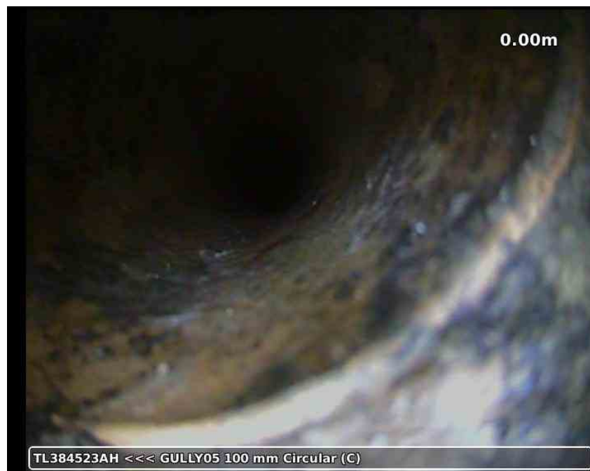
20210617-183433-snap0001.jpg, 00:00:02, 0.00 m Water level, 5% % of the vertical dimension
