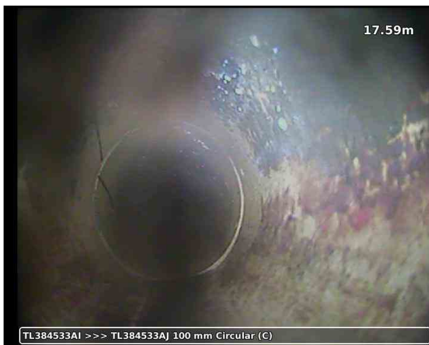
20210617-191337-snap0015.jpg, 00:05:00, 17.59 m Roots, fine at joint
