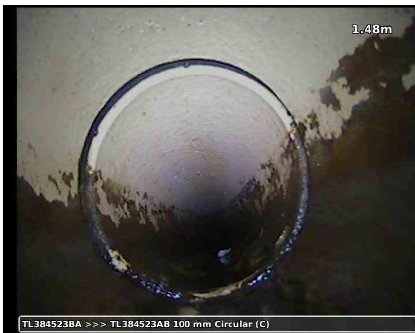
20210617-164942-snap0005.jpg, 00:00:52, 1.48 m Open joint, medium
