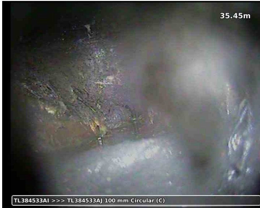
20210617-191337-snap0026.jpg, 00:08:48, 35.45 m Finish node type, manhole, reference number: TL384533AJ, HIDDEN CHAMBER
