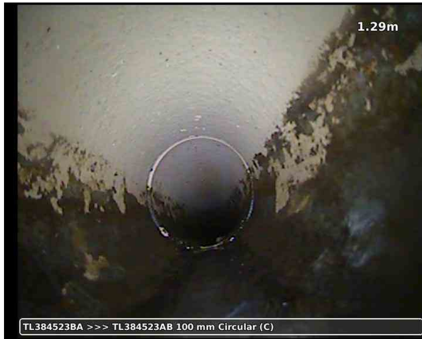
20210617-164942-snap0004.jpg, 00:00:40, 1.29 m Attached deposits, fouling, from 02 to 10 o'clock, 5% % cross-sectional area loss, S02
