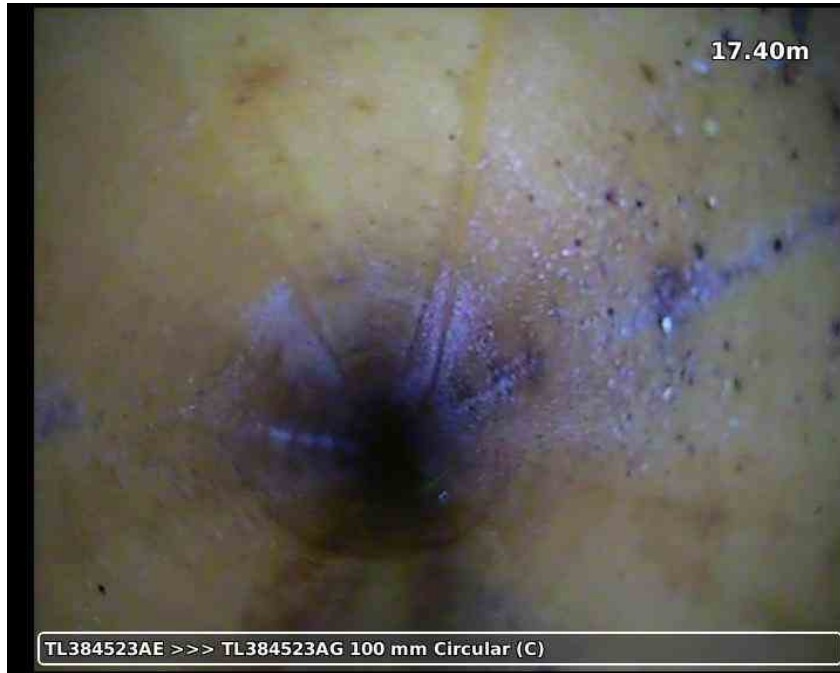
20210617-181934-snap0012.jpg, 00:03:34, 17.40 m Water level, 5% % of the vertical dimension
