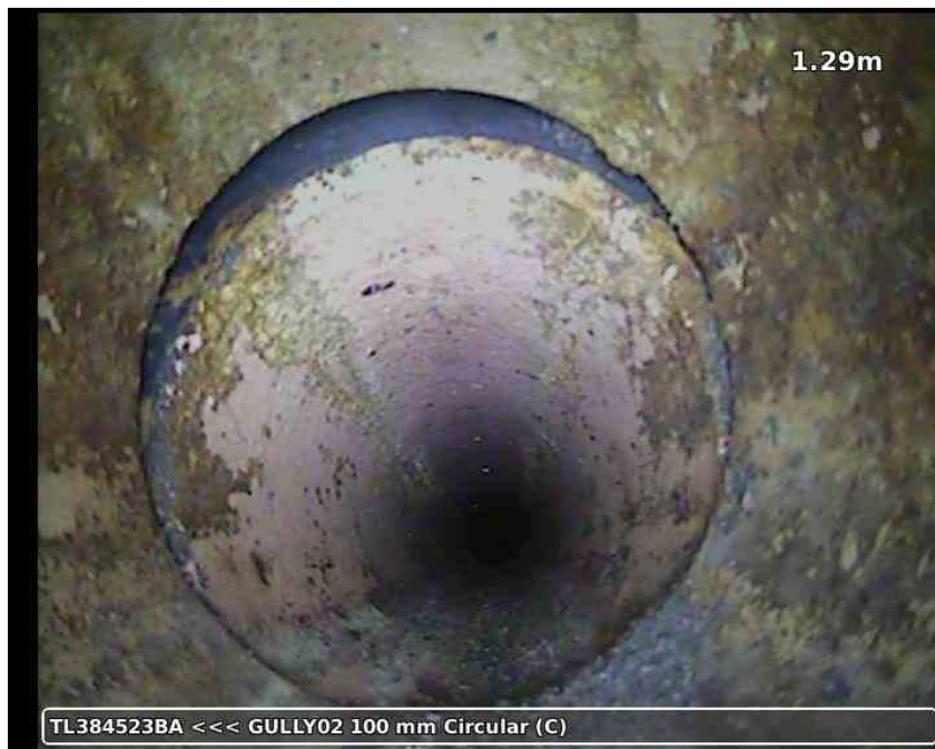
20210617-164707-snap0003.jpg, 00:00:35, 1.29 m Open joint, medium
