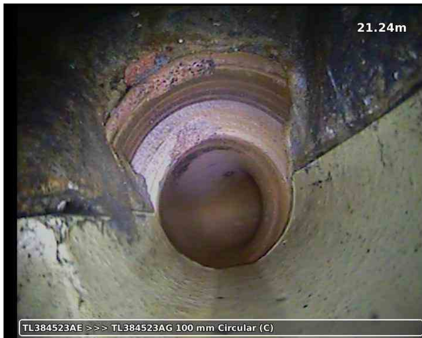
20210617-181934-snap0013.jpg, 00:04:08, 21.24 m Finish node type, manhole, reference number: TL384523AG
