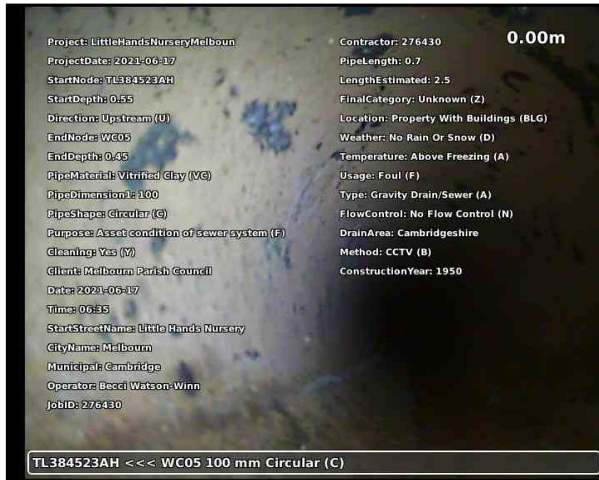
20210617-183609-snap0000.jpg, 00:00:00, 0.00 m Start node type, manhole, reference number: TL384523AH
