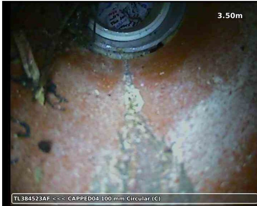
20210617-180144-snap0006.jpg, 00:01:38, 3.50 m Finish node type, other special chamber, reference number: CAPPED04, Internal rest bend CAPPED04
