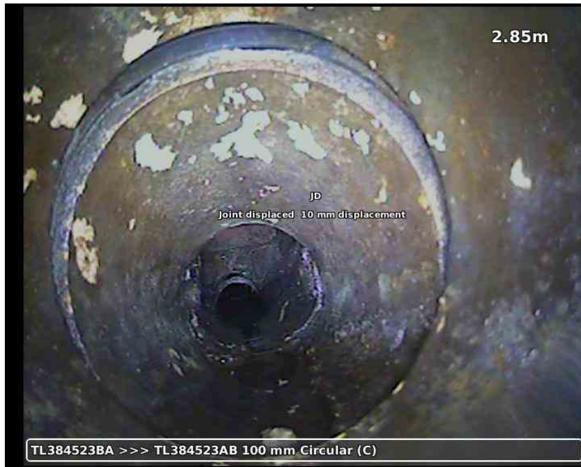
20210617-164942-snap0008.jpg, 00:01:21, 2.85 m Open joint, medium
