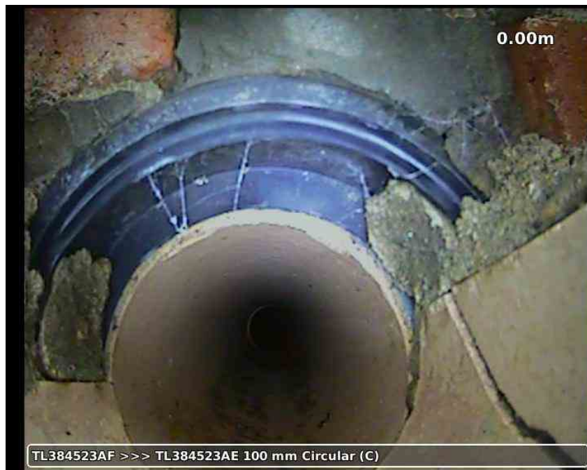
20210617-180721-snap0001.jpg, 00:00:01, 0.00 m Water level, 0% % of the vertical dimension, DISUSED LINE FROM PUBLIC TOILETS
