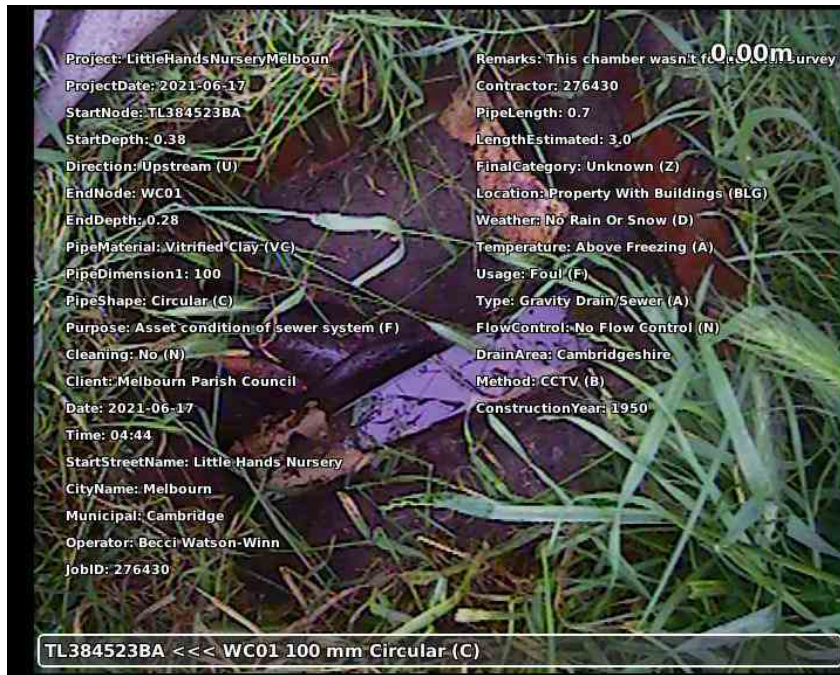
20210617-164432-snap0000.jpg, 00:00:00, 0.00 m Start node type, manhole, reference number: TL384523BA
