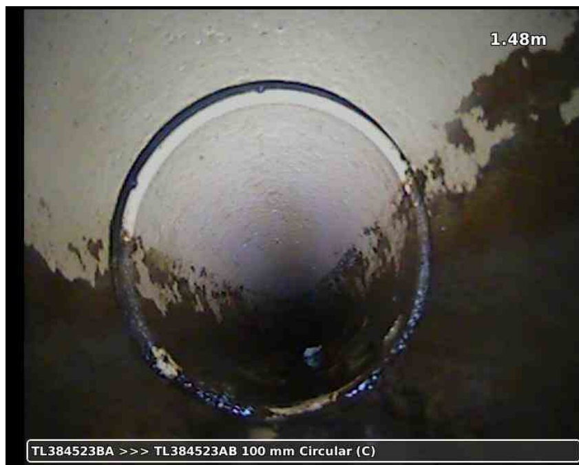
20210617-164942-snap0005.jpg, 00:00:52, 1.48 m Open joint, medium
