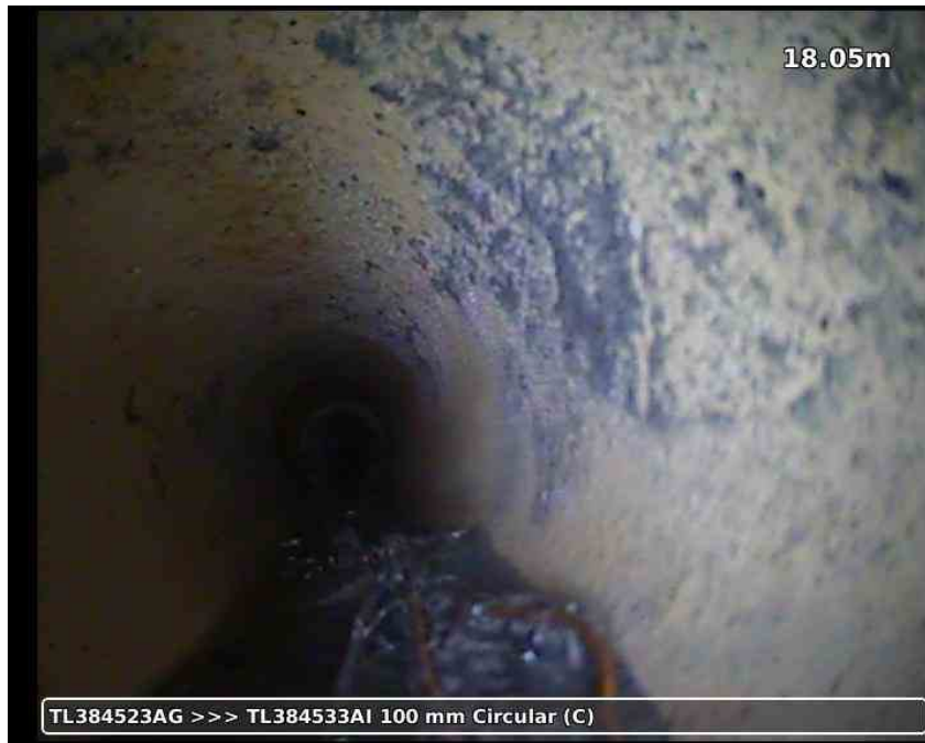
20210617-185600-snap0022.jpg, 00:04:28, 18.05 m Roots, mass, 20% % cross-sectional area loss
