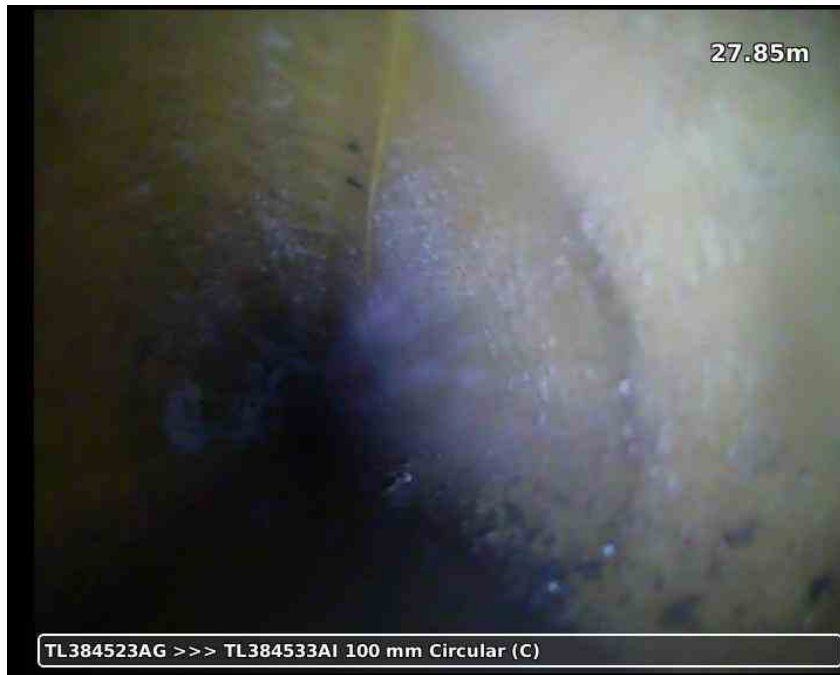
20210617-185600-snap0030.jpg, 00:06:38, 27.85 m Water level, 10% % of the vertical dimension
