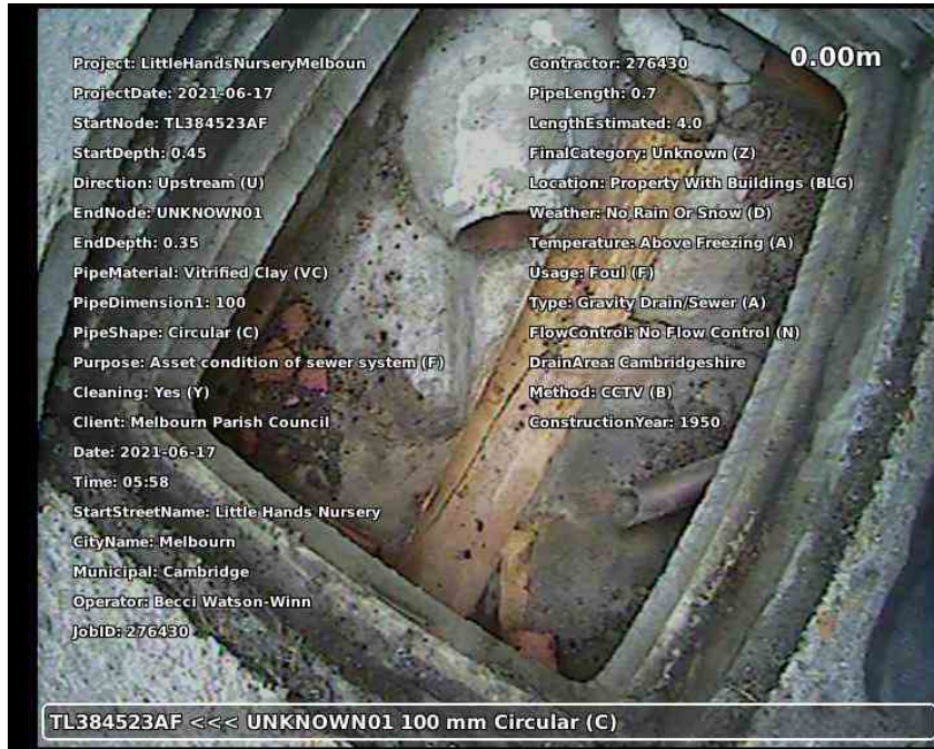
20210617-175837-snap0000.jpg, 00:00:01, 0.00 m Start node type, manhole, reference number: TL384523AF
