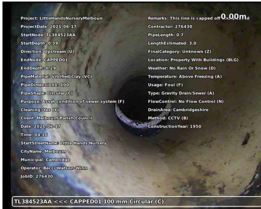
20210617-161651-snap0000.jpg, 00:00:00, 0.00 m Start node type, manhole, reference number: TL384523AA
