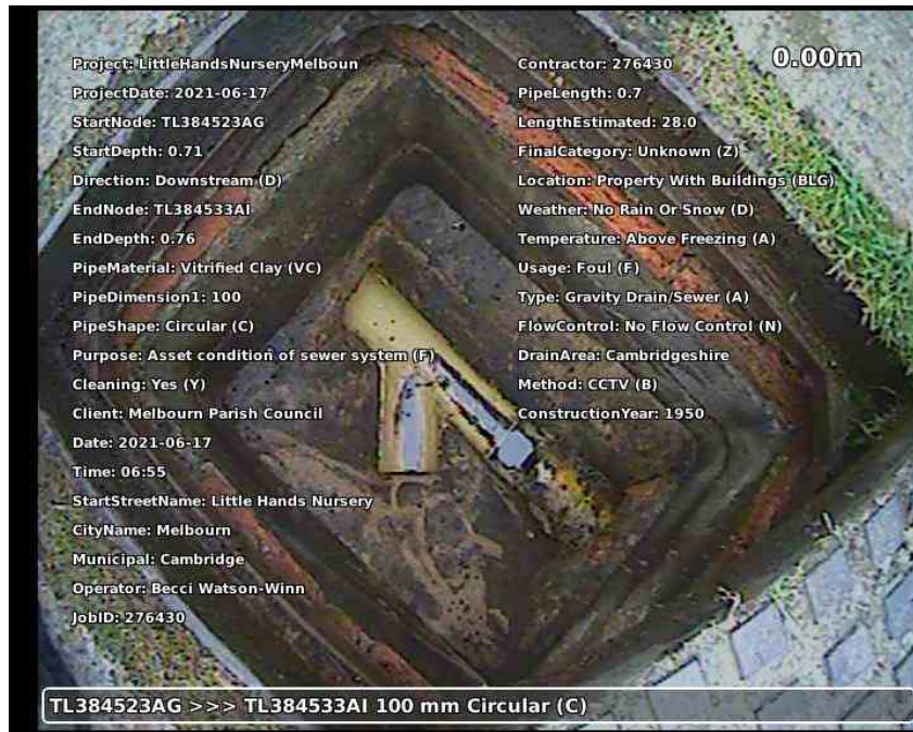
20210617-185600-snap0000.jpg, 00:00:03, 0.00 m Start node type, manhole, reference number: TL384523AG
