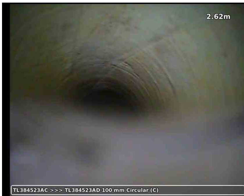
20210617-171630-snap0006.jpg, 00:01:46, 2.62 m Water level, 50% % of the vertical dimension
