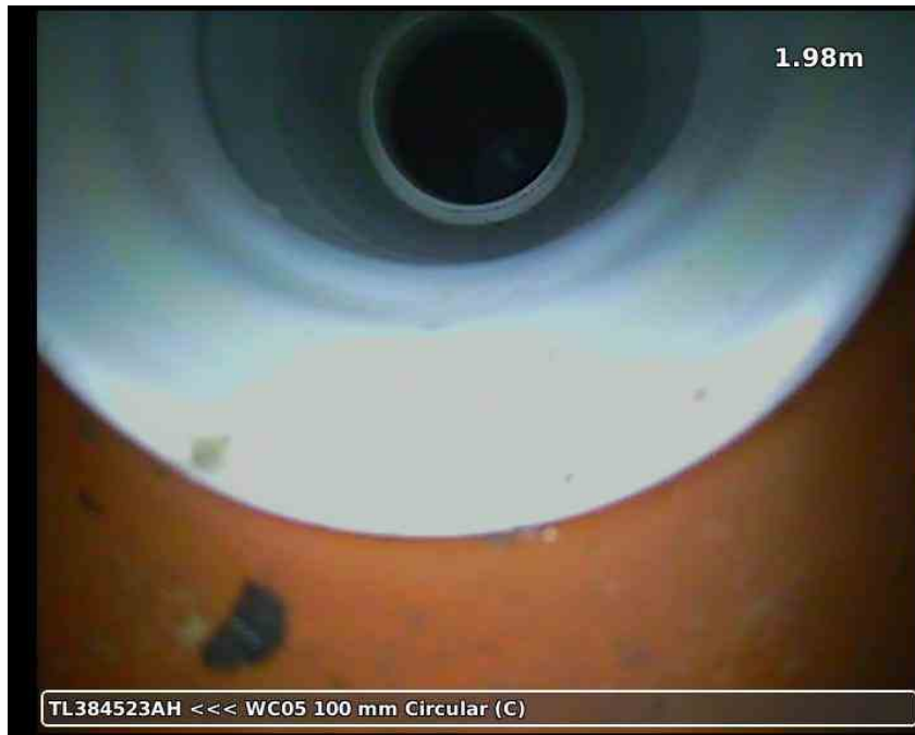
20210617-183609-snap0002.jpg, 00:00:25, 1.98 m Finish node type, other special chamber, reference number: WC05, Internal rest bend WC05
