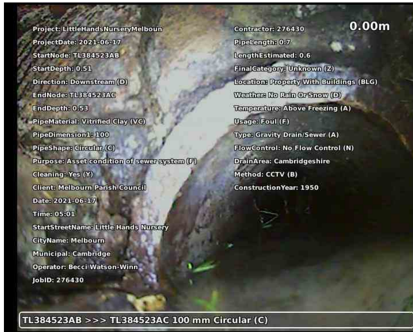
20210617-170147-snap0000.jpg, 00:00:01, 0.00 m Start node type, manhole, reference number: TL384523AB
