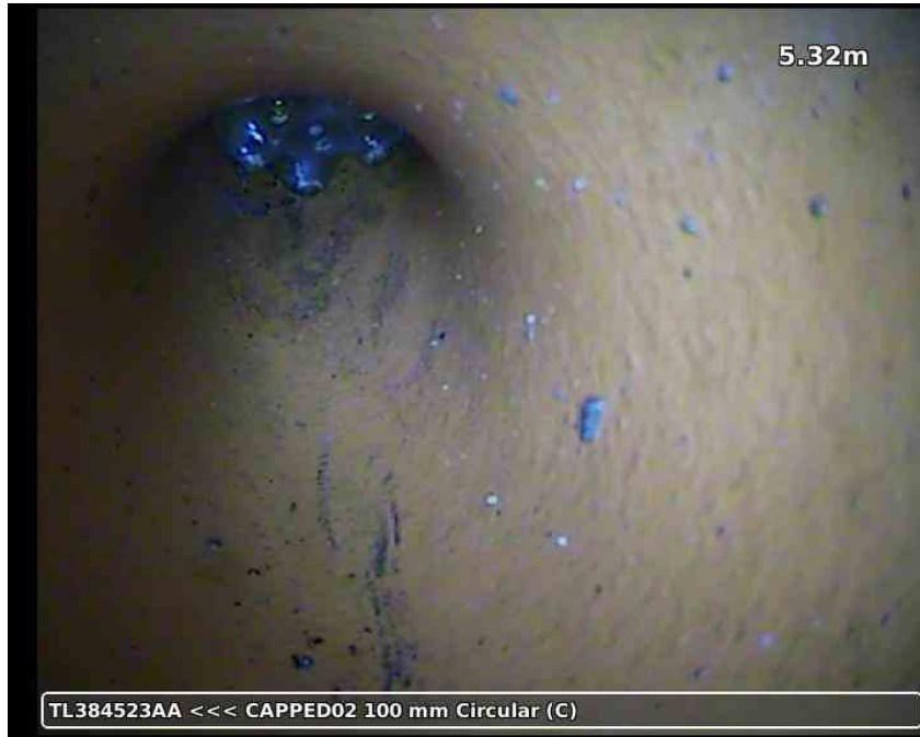
20210617-161854-snap0004.jpg, 00:01:40, 5.32 m Finish node type, other special chamber, reference number: CAPPED02, Internal rest bend CAPPED OFF
