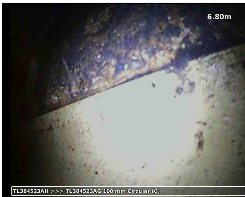
20210617-184209-snap0007.jpg, 00:01:39, 6.80 m Finish node type, manhole, reference number: TL384523AG
