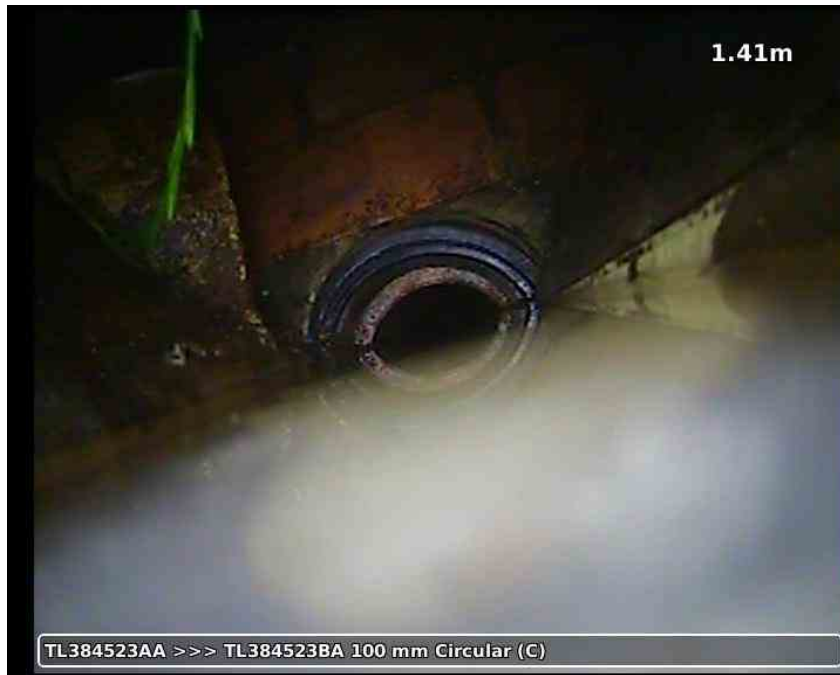
20210617-163005-snap0006.jpg, 00:01:02, 1.41 m Water level, 40% % of the vertical dimension
