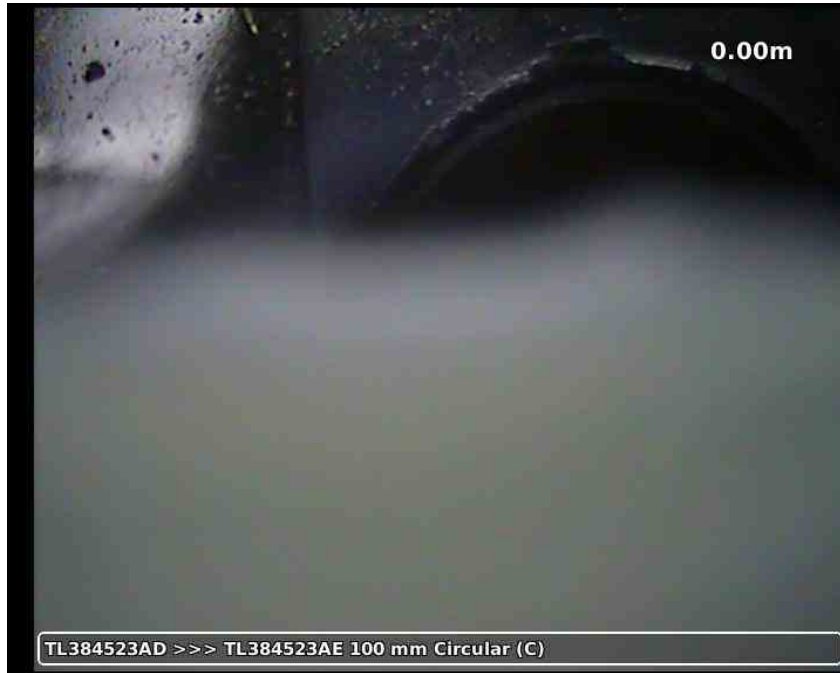
20210617-173215-snap0000.jpg, 00:00:01, 0.00 m Start node type, manhole, reference number: TL384523AD
