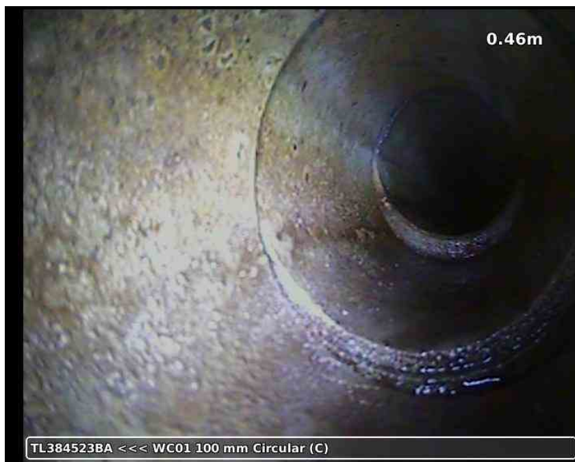
20210617-164432-snap0005.jpg, 00:00:35, 0.46 m Open joint, medium
