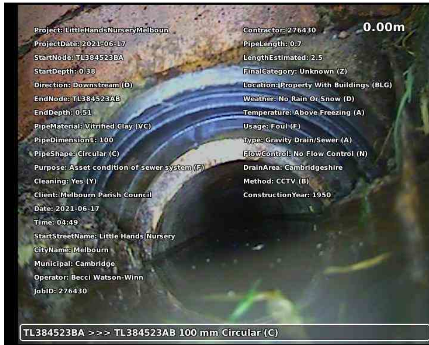
20210617-164942-snap0000.jpg, 00:00:00, 0.00 m Start node type, manhole, reference number: TL384523BA
