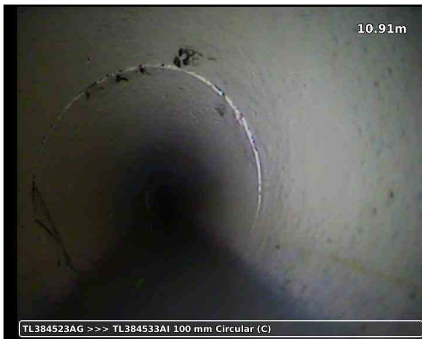
20210617-185600-snap0017.jpg, 00:03:18, 10.91 m Roots, fine, ENTERING THROUGH FC
