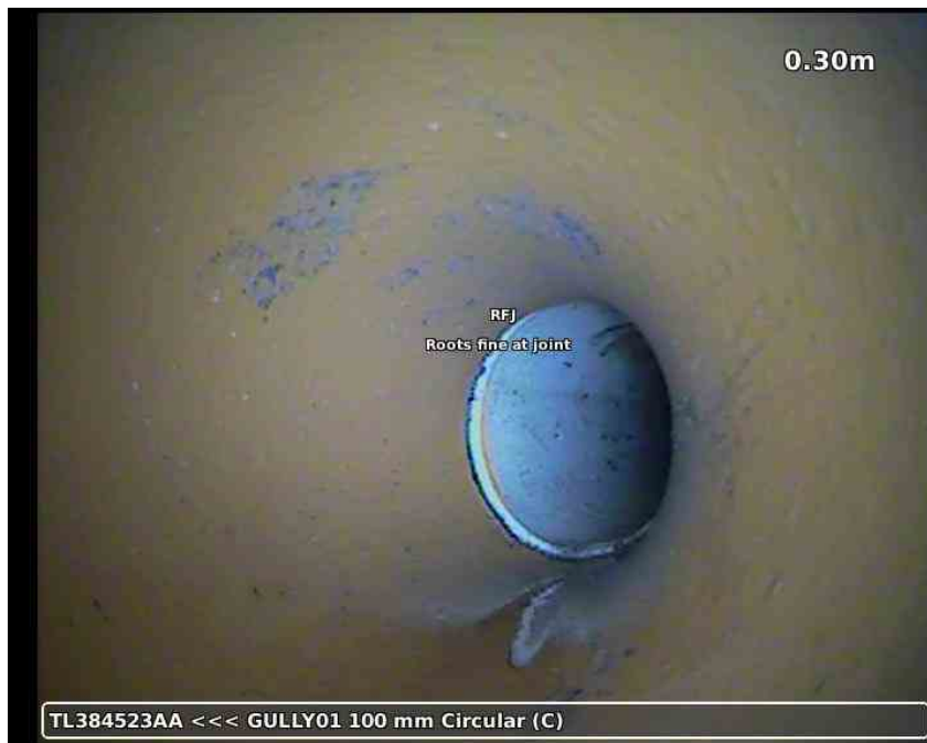
20210617-161336-snap0003.jpg, 00:00:17, 0.30 m Line deviates right
