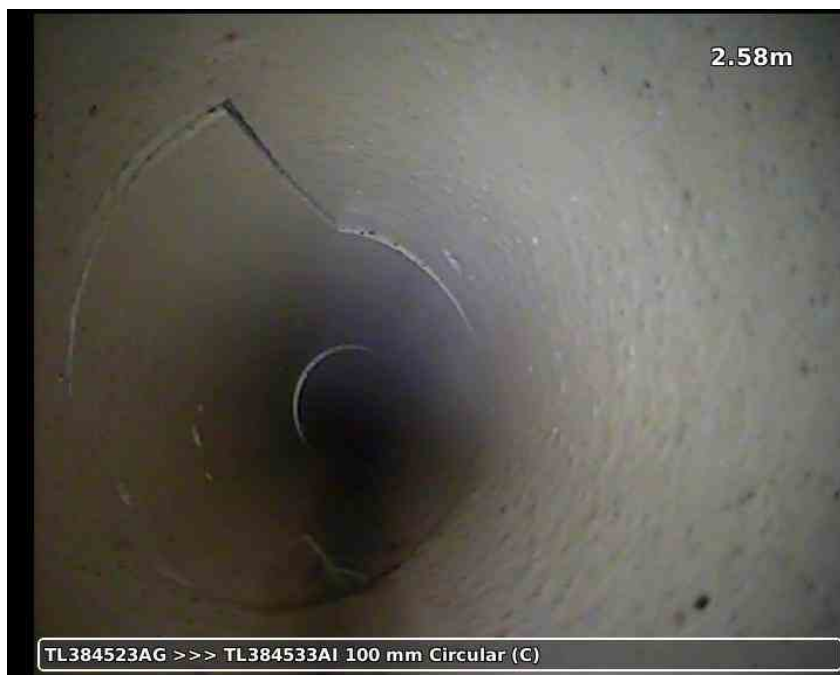
20210617-185600-snap0007.jpg, 00:01:12, 2.58 m Fracture spiral, from 12 to 11 o'clock
