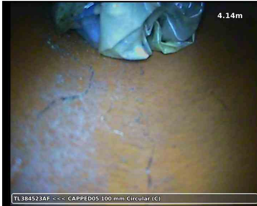
20210617-180419-snap0004.jpg, 00:01:03, 4.14 m Finish node type, other special chamber, reference number: CAPPED05, Internal rest bend CAPPED OFF
