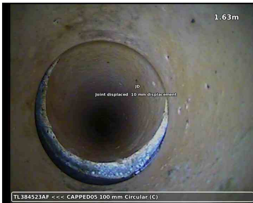
20210617-180419-snap0003.jpg, 00:00:40, 1.63 m Open joint, medium
