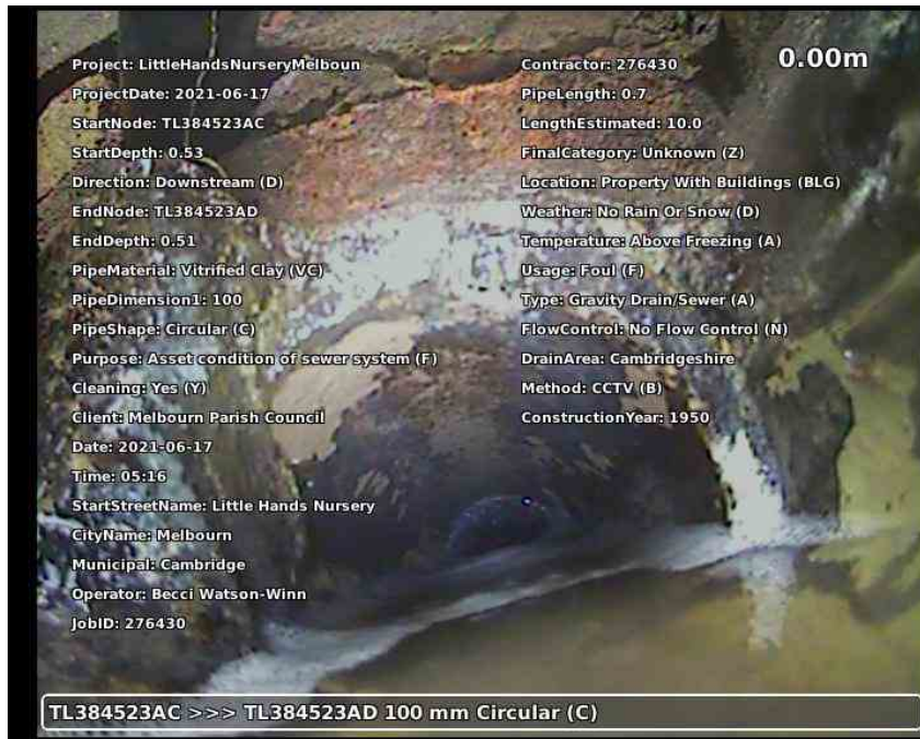
20210617-171630-snap0000.jpg, 00:00:01, 0.00 m Start node type, manhole, reference number: TL384523AC
