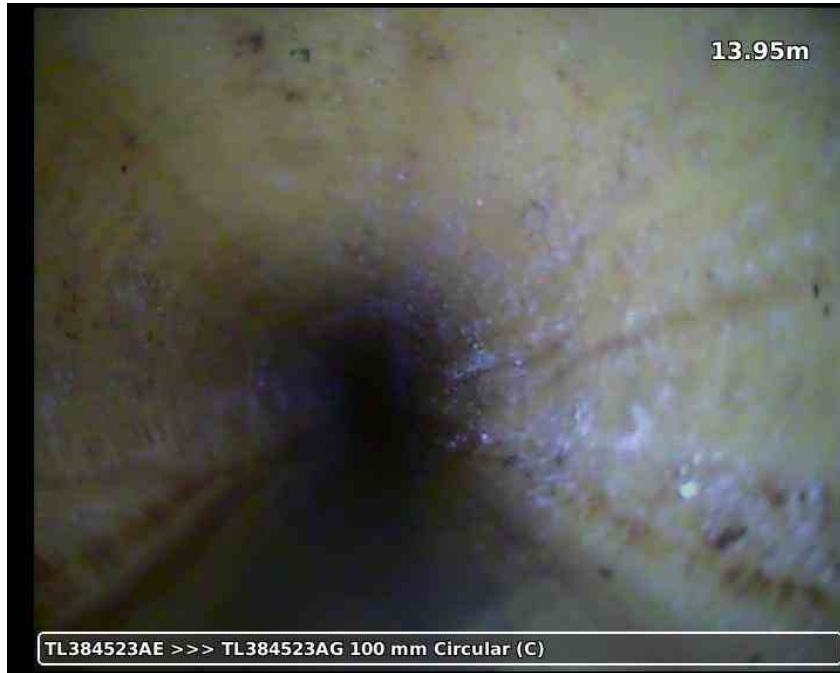
20210617-181934-snap0010.jpg, 00:02:53, 13.95 m Water level, 10% % of the vertical dimension
