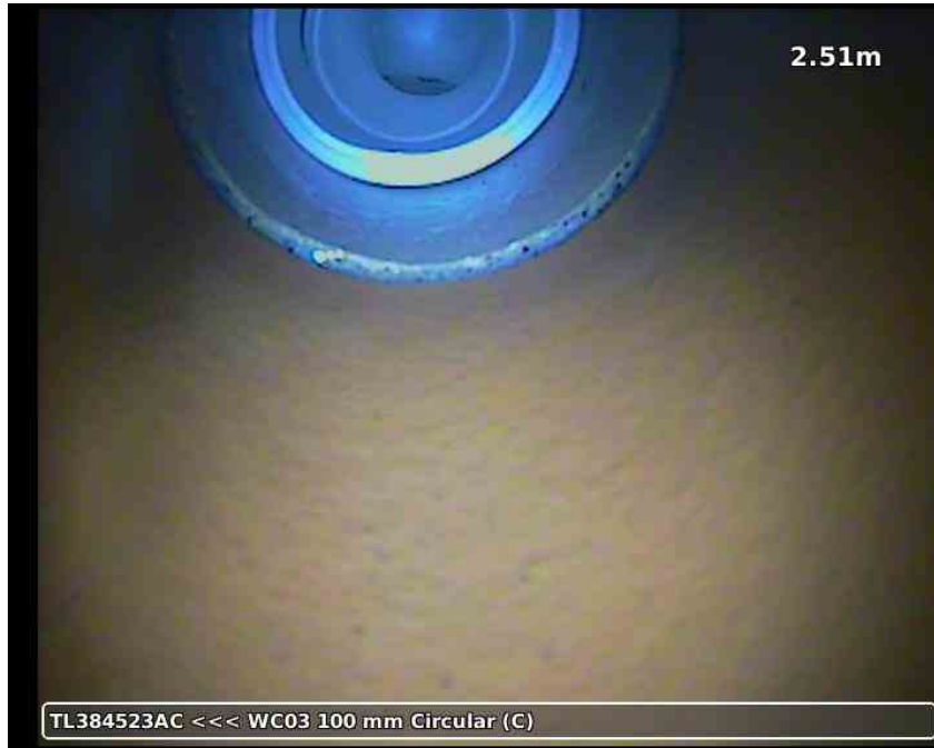
20210617-171046-snap0006.jpg, 00:01:00, 2.51 m Finish node type, other special chamber, reference number: WC03, Internal rest bend WC03
