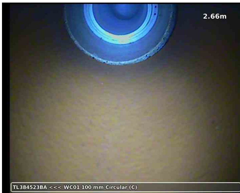
20210617-164432-snap0007.jpg, 00:01:15, 2.66 m Finish node type, other special chamber, reference number: WC01, Internal rest bend WC01
