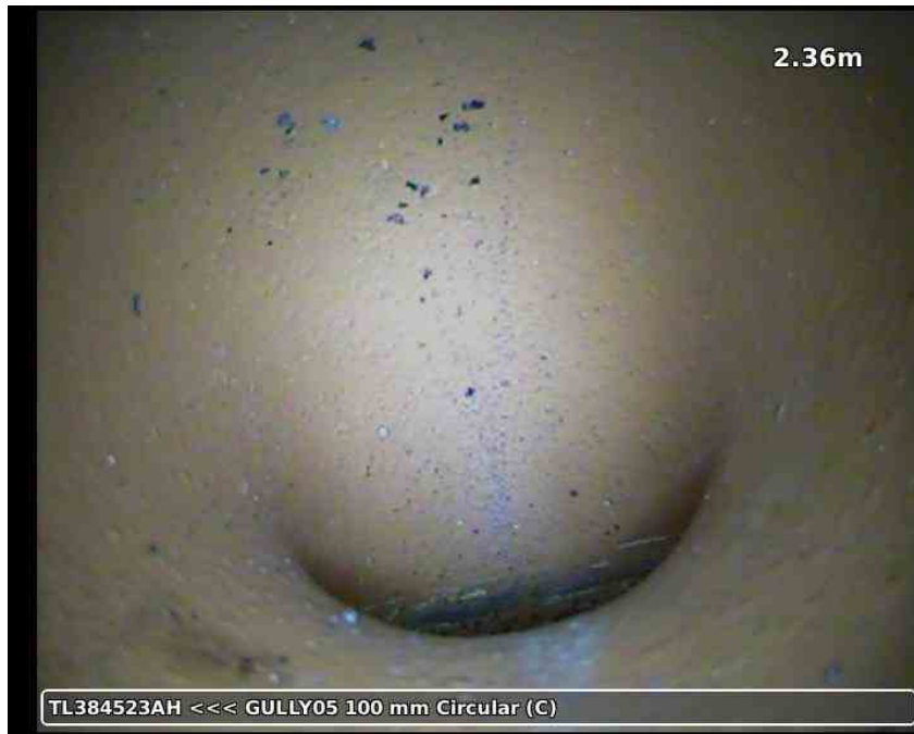
20210617-183433-snap0002.jpg, 00:00:35, 2.36 m Finish node type, gully, reference number: GULLY05, Internal gully
