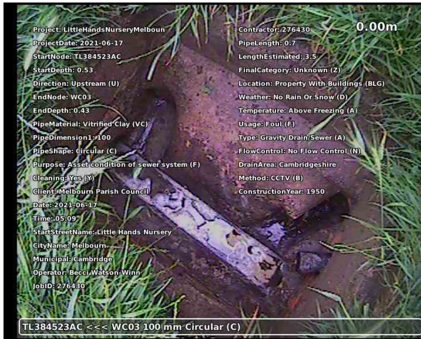
20210617-171046-snap0000.jpg, 00:00:01, 0.00 m Start node type, manhole, reference number: TL384523AC
