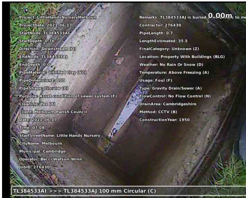
20210617-191337-snap0000.jpg, 00:00:01, 0.00 m Start node type, manhole, reference number: TL384533AI
