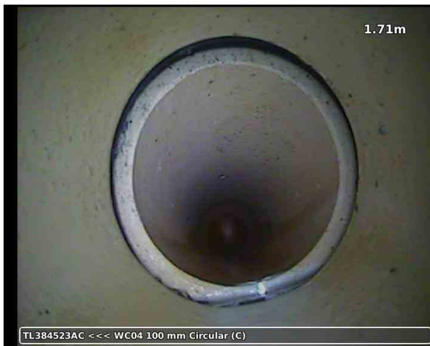
20210617-171300-snap0003.jpg, 00:00:29, 1.71 m Open joint, medium
