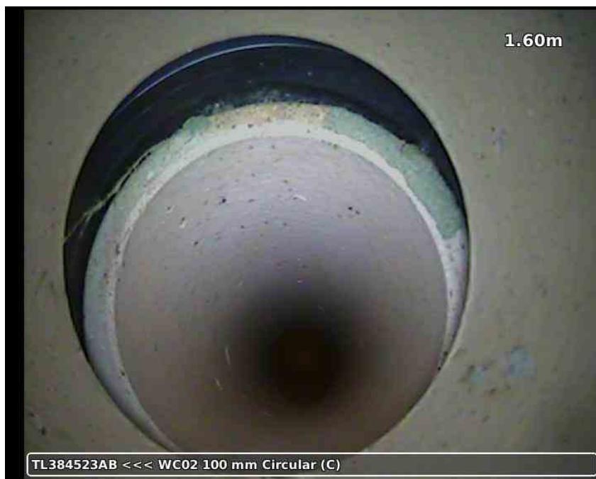
20210617-165855-snap0003.jpg, 00:00:36, 1.60 m Open joint, large
