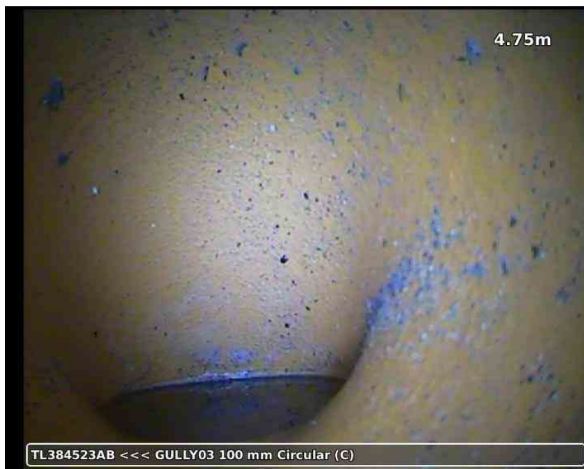
20210617-165624-snap0003.jpg, 00:00:56, 4.75 m Finish node type, gully, reference number: GULLY03, Internal gully
