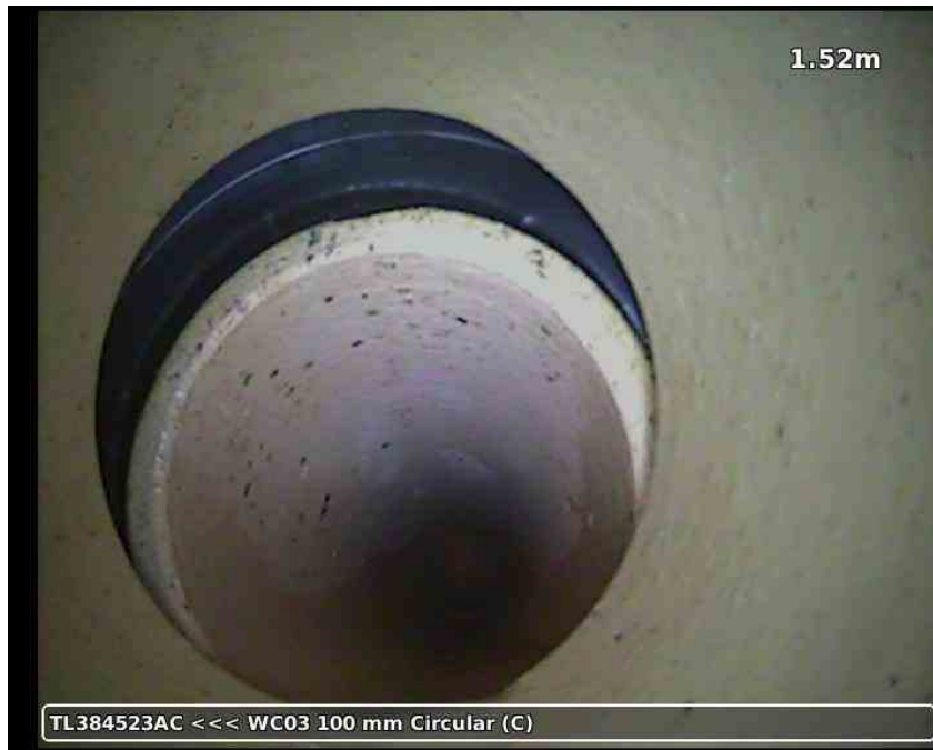
20210617-171046-snap0002.jpg, 00:00:23, 1.52 m Open joint, large
