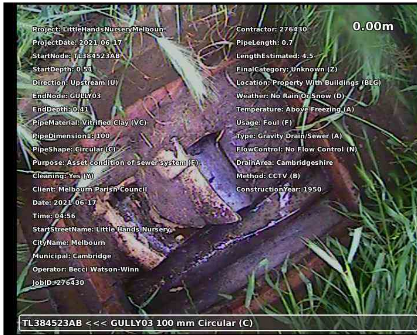
20210617-165624-snap0000.jpg, 00:00:00, 0.00 m Start node type, manhole, reference number: TL384523AB
