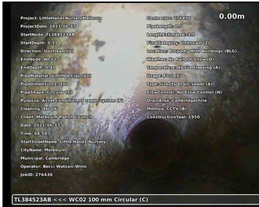
20210617-165855-snap0000.jpg, 00:00:00, 0.00 m Start node type, manhole, reference number: TL384523AB
