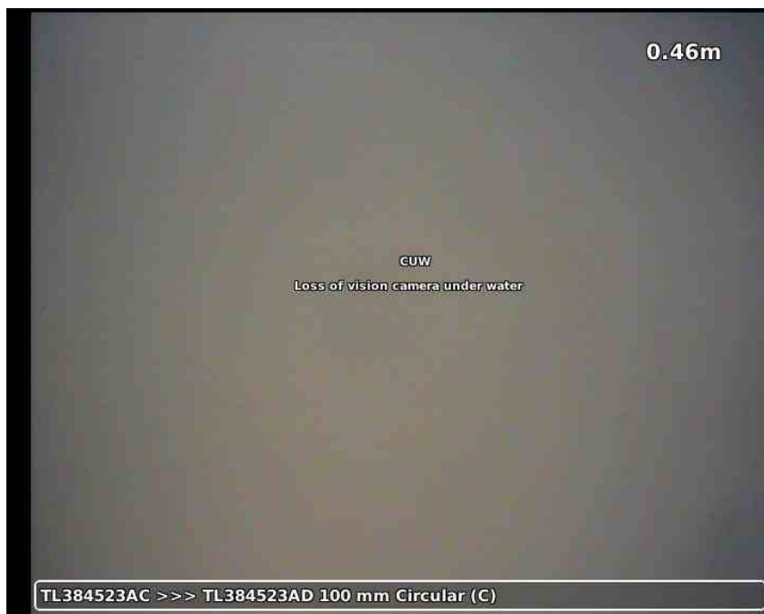
20210617-171630-snap0003.jpg, 00:00:33, 0.46 m Loss of vision, camera under water, S01
