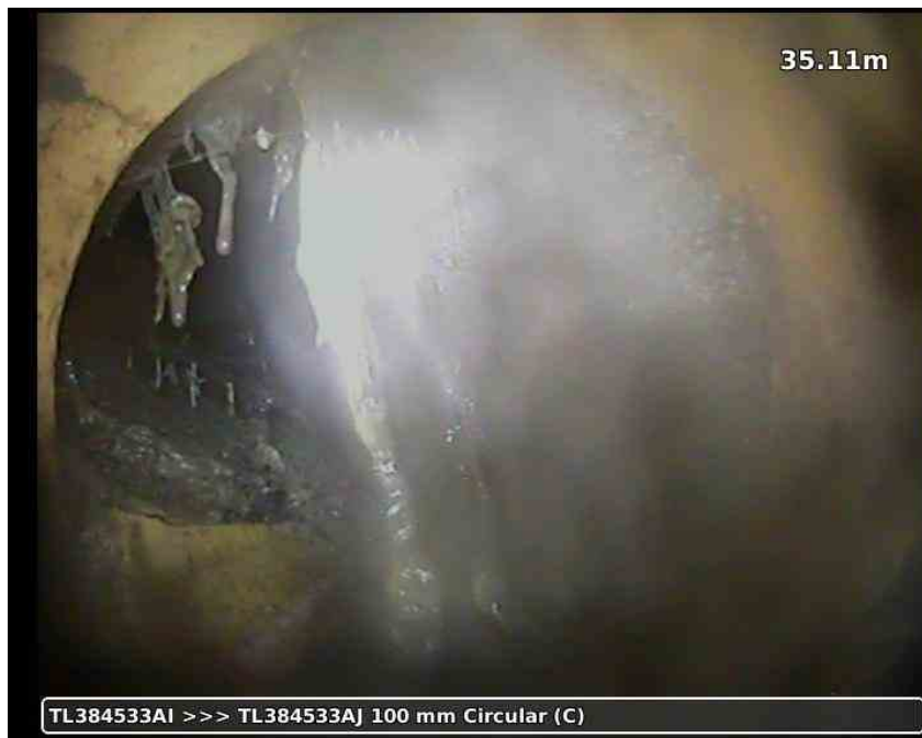
20210617-191337-snap0025.jpg, 00:08:34, 35.11 m Roots, mass, 30% % cross-sectional area loss
