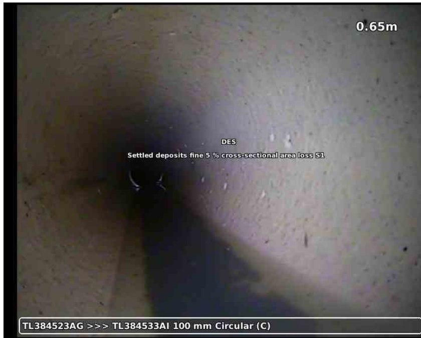
20210617-185600-snap0004.jpg, 00:00:24, 0.65 m Water level, 10% % of the vertical dimension
