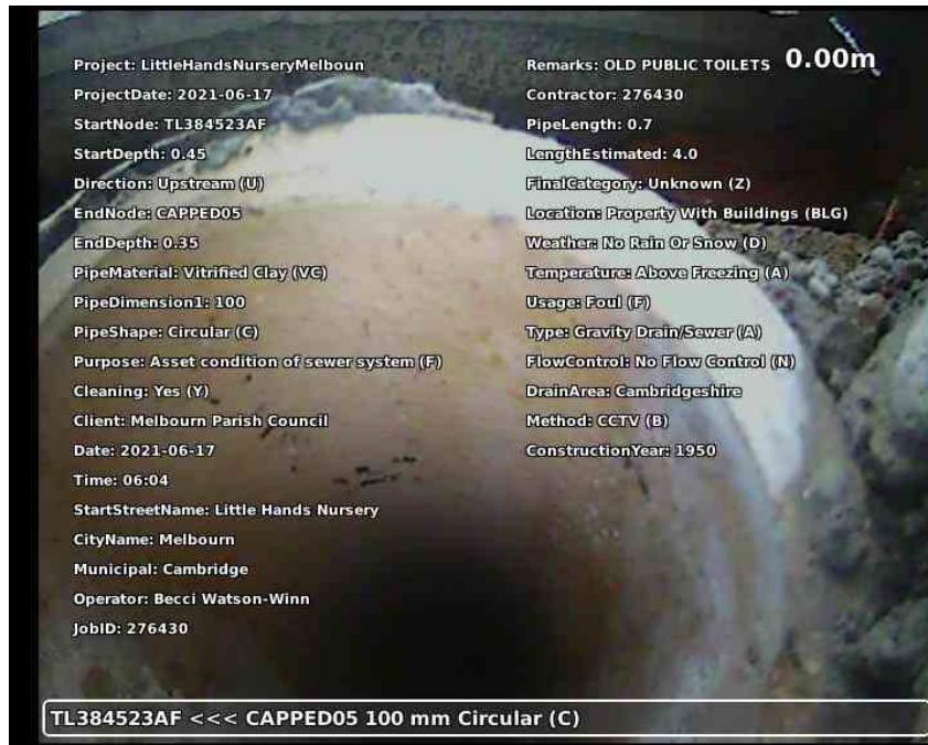
20210617-180419-snap0000.jpg, 00:00:00, 0.00 m Start node type, manhole, reference number: TL384523AF
