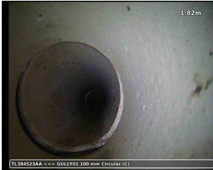
20210617-161336-snap0004.jpg, 00:00:31, 1.82 m Open joint, medium
