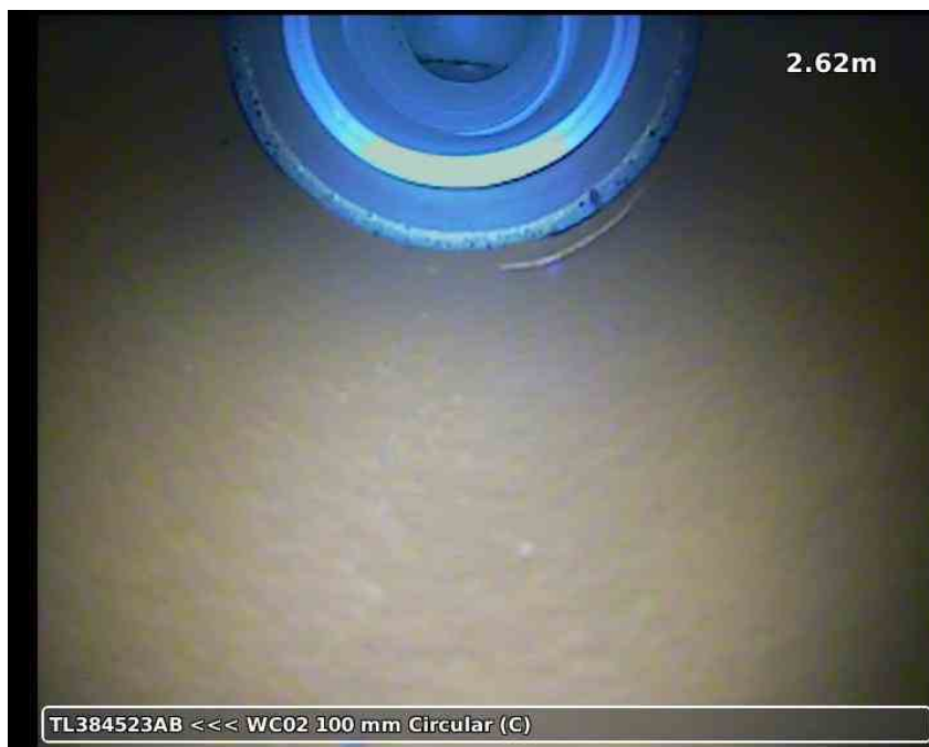
20210617-165855-snap0005.jpg, 00:01:01, 2.62 m Finish node type, other special chamber, reference number: WC02, Internal rest bend WC02
