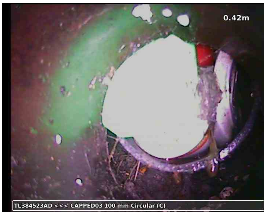
20210617-172705-snap0003.jpg, 00:00:48, 0.42 m Finish node type, other special chamber, reference number: CAPPED03, CAPPED OFF LINE
