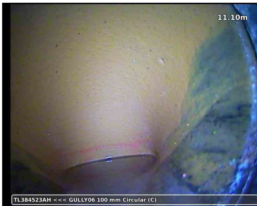
20210617-183738-snap0007.jpg, 00:02:07, 11.10 m Finish node type, gully, reference number: GULLY06, Internal gully
