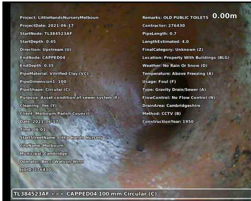
20210617-180144-snap0000.jpg, 00:00:00, 0.00 m Start node type, manhole, reference number: TL384523AF
