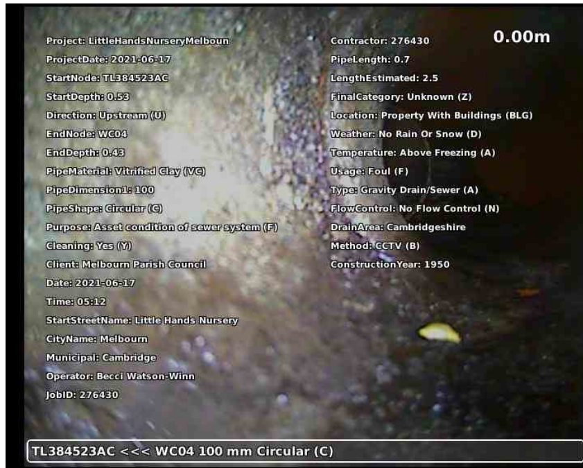
20210617-171300-snap0000.jpg, 00:00:00, 0.00 m Start node type, manhole, reference number: TL384523AC
