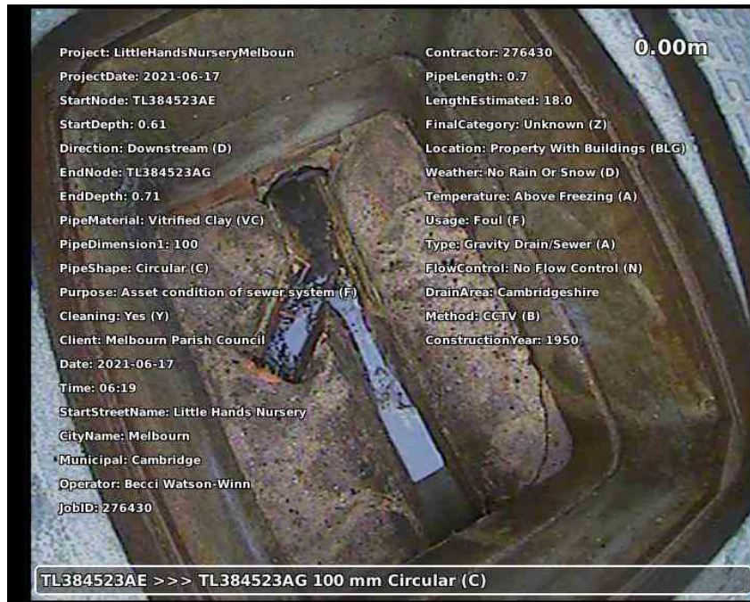
20210617-181934-snap0000.jpg, 00:00:01, 0.00 m Start node type, manhole, reference number: TL384523AE
