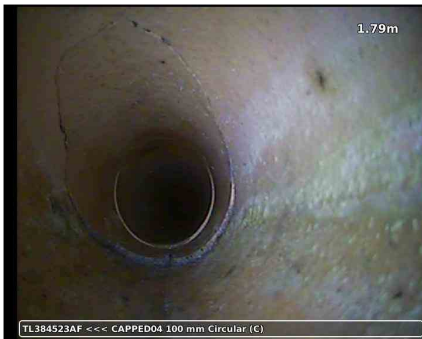
20210617-180144-snap0005.jpg, 00:01:11, 1.79 m Fracture spiral, from 12 to 11 o'clock
