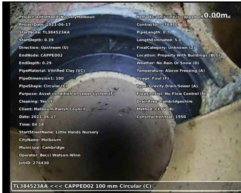
20210617-161854-snap0000.jpg, 00:00:00, 0.00 m Start node type, manhole, reference number: TL384523AA
