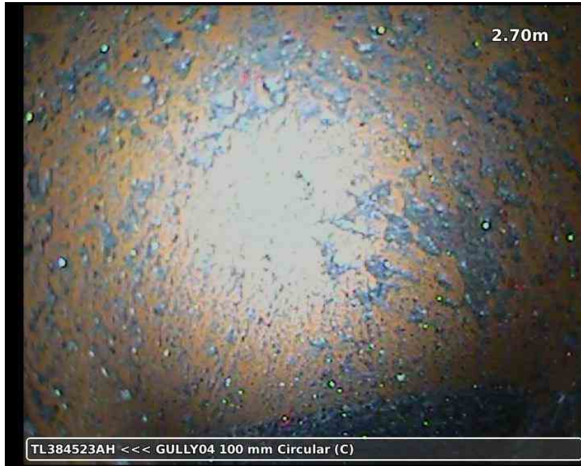
20210617-183231-snap0004.jpg, 00:00:37, 2.70 m Finish node type, gully, reference number: GULLY04, Internal gully
