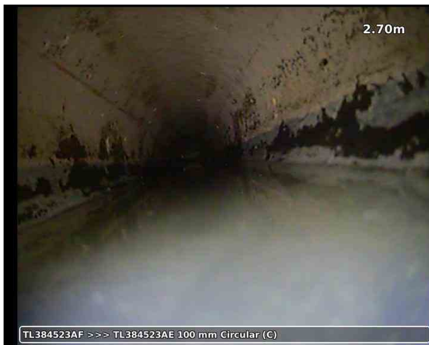
20210617-180721-snap0003.jpg, 00:00:52, 2.70 m Water level, 25% % of the vertical dimension
