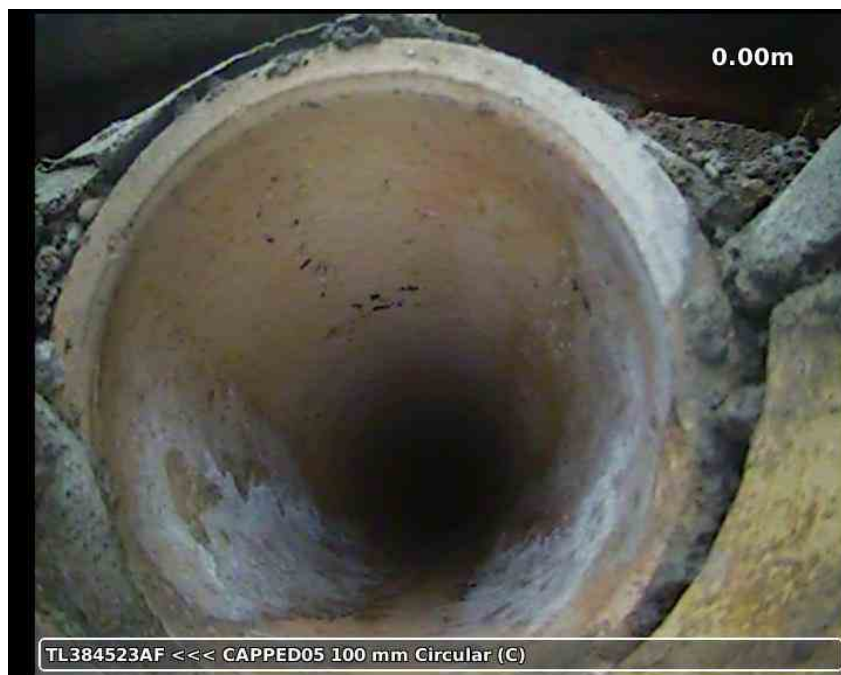
20210617-180419-snap0001.jpg, 00:00:02, 0.00 m Water level, 0% % of the vertical dimension, CAPPED OFF
