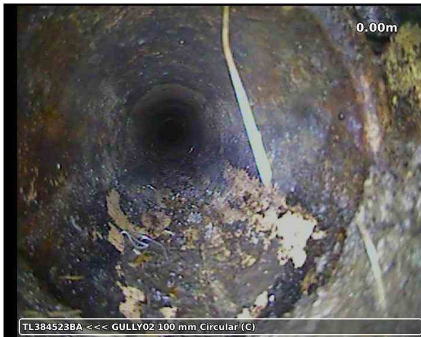
20210617-164707-snap0001.jpg, 00:00:01, 0.00 m Water level, 0% % of the vertical dimension, DISUSED GULLY
