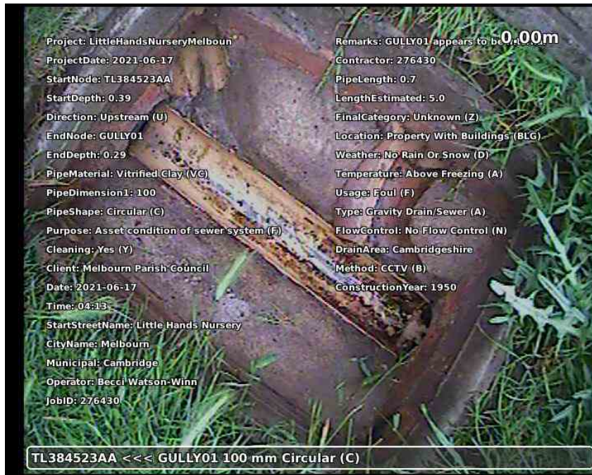
20210617-161336-snap0000.jpg, 00:00:00, 0.00 m Start node type, manhole, reference number: TL384523AA
