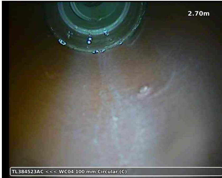
20210617-171300-snap0004.jpg, 00:00:43, 2.70 m Finish node type, other special chamber, reference number: WC04, Internal rest bend WC04
