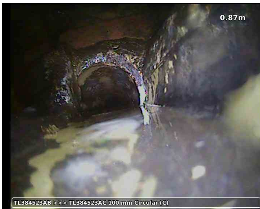
20210617-170147-snap0003.jpg, 00:00:29, 0.87 m Water level, 20% % of the vertical dimension, BACK FLOWING
