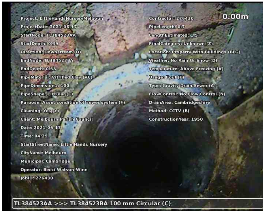
20210617-163005-snap0000.jpg, 00:00:00, 0.00 m Start node type, manhole, reference number: TL384523AA
