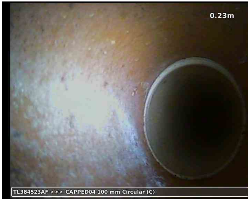
20210617-180144-snap0002.jpg, 00:00:15, 0.23 m Line deviates right
