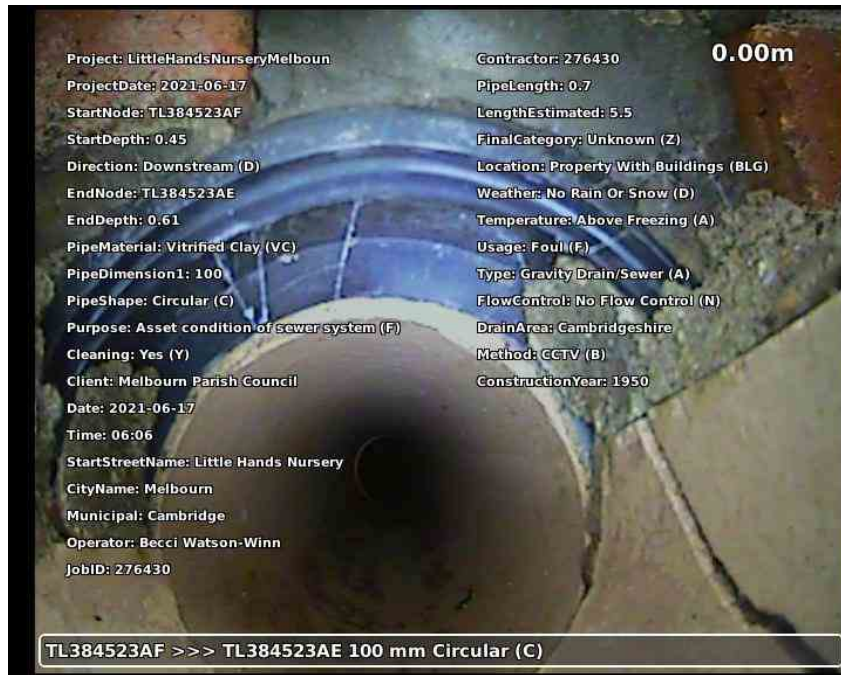
20210617-180721-snap0000.jpg, 00:00:00, 0.00 m Start node type, manhole, reference number: TL384523AF
