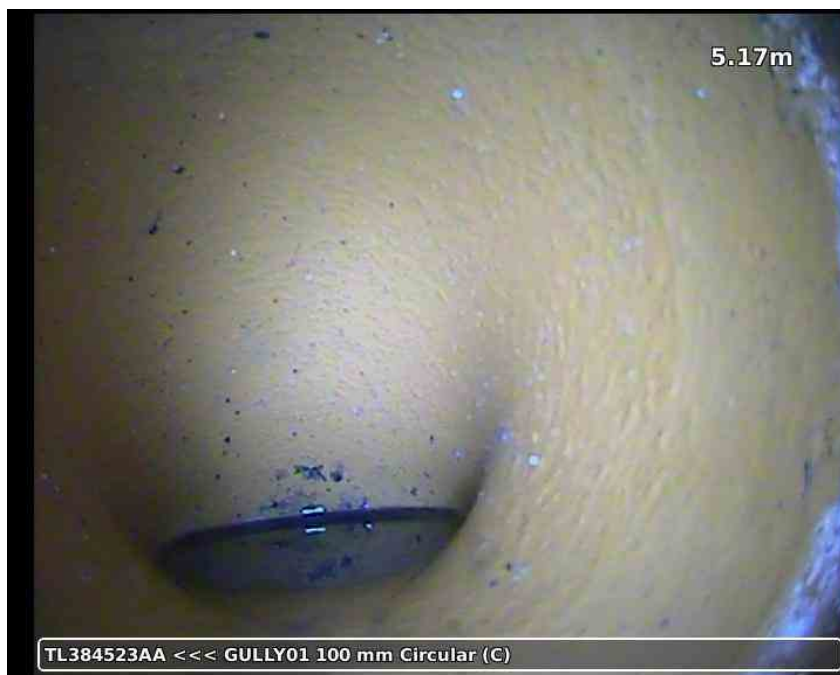
20210617-161336-snap0005.jpg, 00:00:56, 5.17 m Finish node type, gully, reference number: GULLY01, Internal gully
