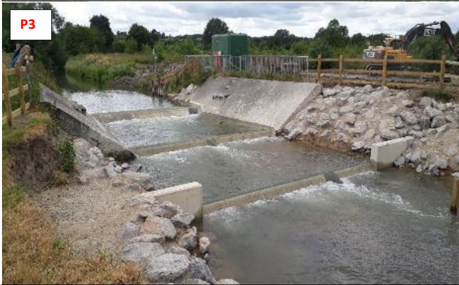
The EA gauging station at Burnt Mill (Haslingfield), July '19 – fish passage has been eased by recent EA work.
