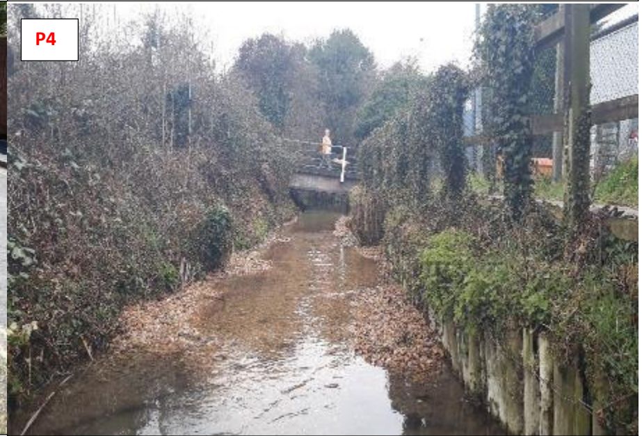
The brook alongside Sainsbury's March 2018 - bed raising with gravel.
