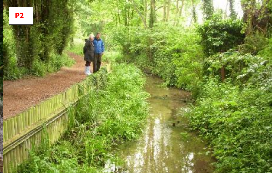
Meldreth May 2012 – the margins have been enhanced through planted brushwood ledges.
