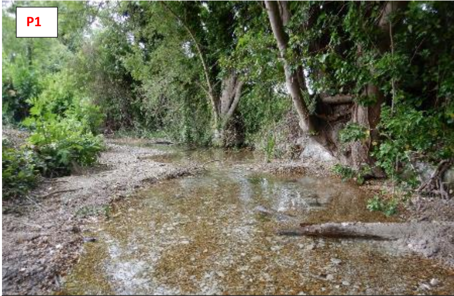
Melbourn playing fields, June 2020 – the bed has been restored with chalk and gravel to increase fish spawning habitat.
