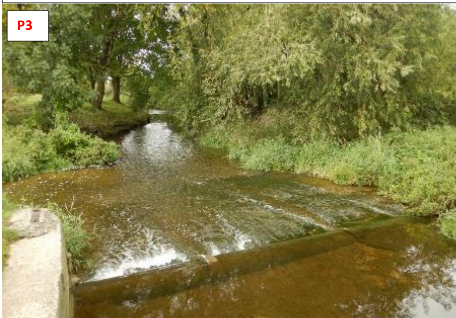
Duxford Aug 2020 – a pipe presents a barrier to fish passage at low-flow.
