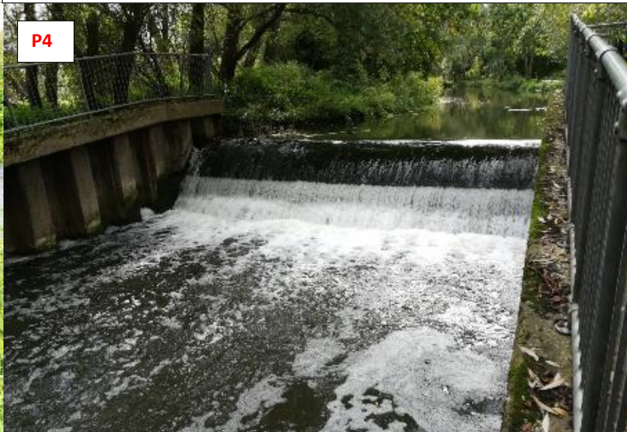
Hauxton Mill, Oct 2020 – weir impounds water and prevents fish passage
