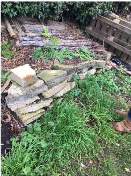
Picture above – bricks/cement to be removed
