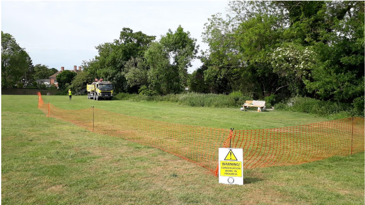
The work area was safely separated from the public.
