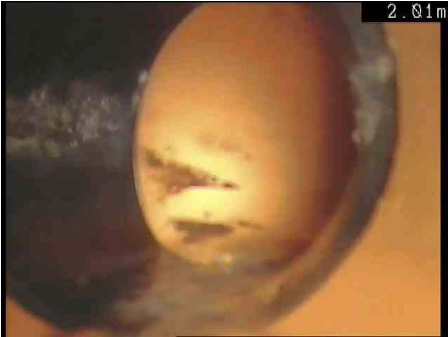
IC5X_f94043d8-51e7-4068-b9f0-39a2bc9f30a7_20181112_095950_928.jpg, 00:00:11, 2.01m Line of sewer deviates right
