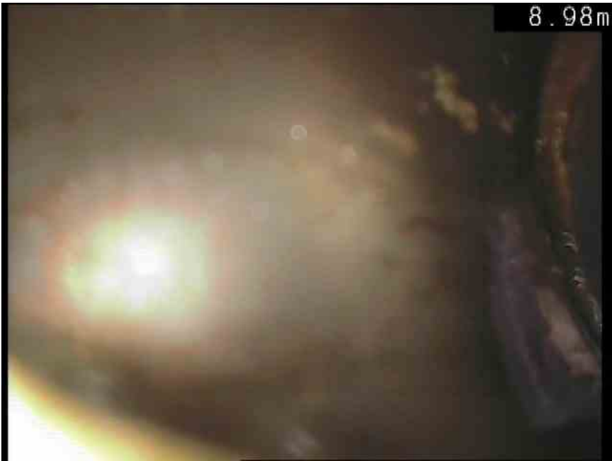
IC3X_c0877a12-83c6-4e64-ac00-31c07757be62_20181112_095537_064.jpg, 00:00:31, 8.98m Line of sewer deviates right
